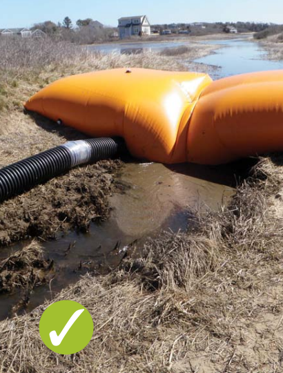
Piped diversion of stream using a bladder bag impervious barrier.
