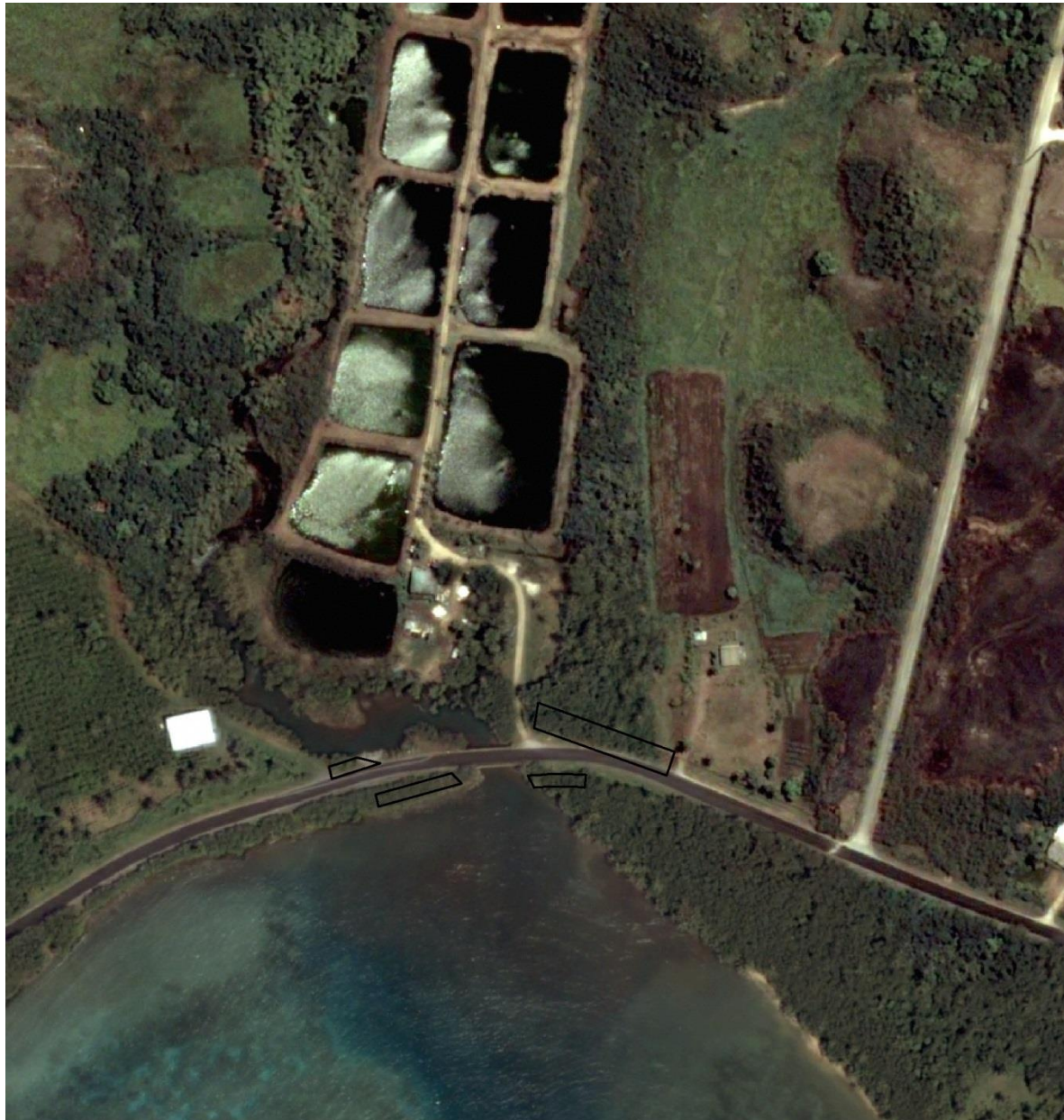
Figure 2. Ajayan Bridge Replacement Project Site
