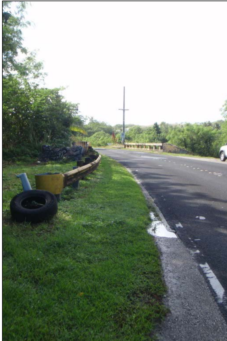
Photo 4 - View from the south east of the Ajayan Bridge
