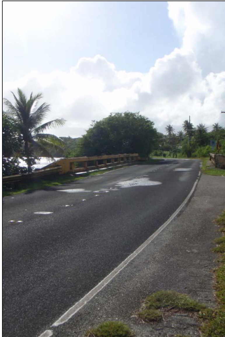
Photo 3 – View from the north and east of the Ajayan Bridge
