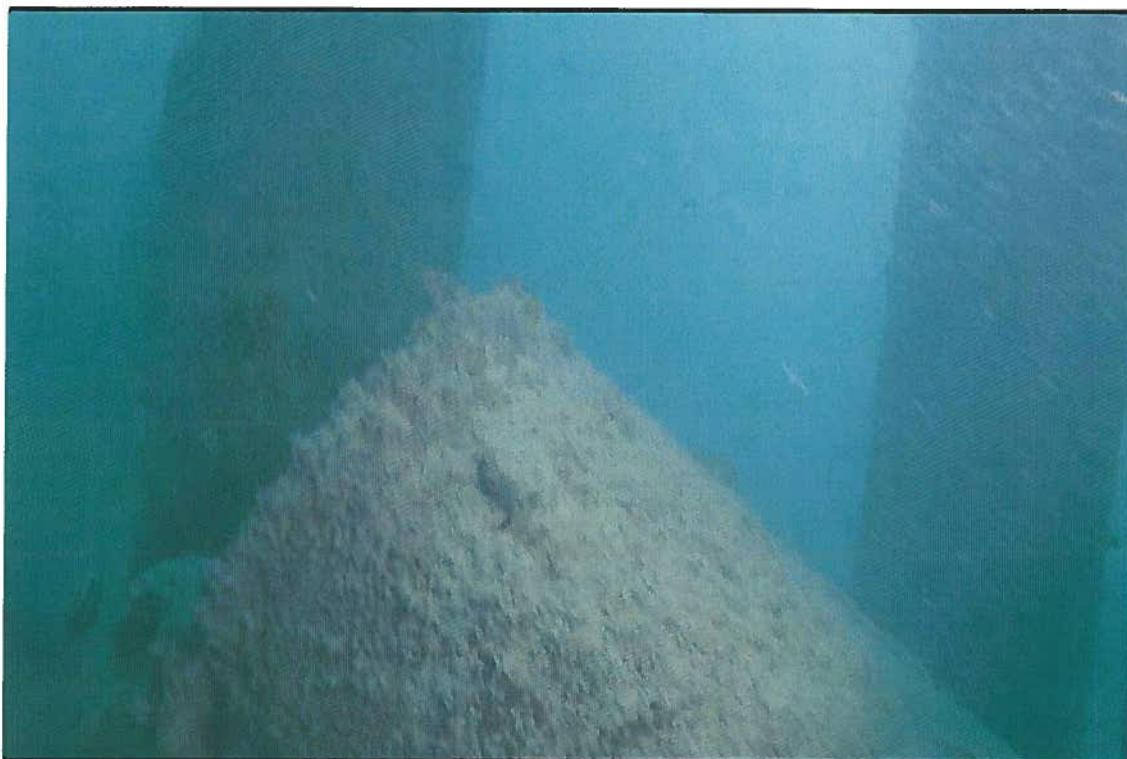
F-1 Dock Piles
