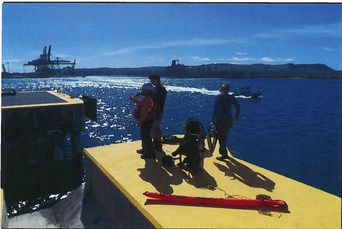
Dive Preparation for F-1 Dock Underwater Inspection
