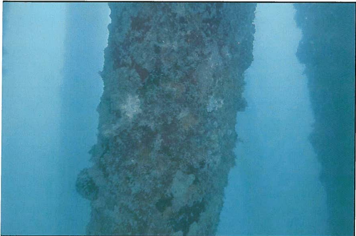
F-1 Dock Piles
