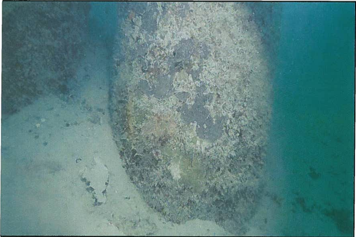
F-1 Dock Piles
