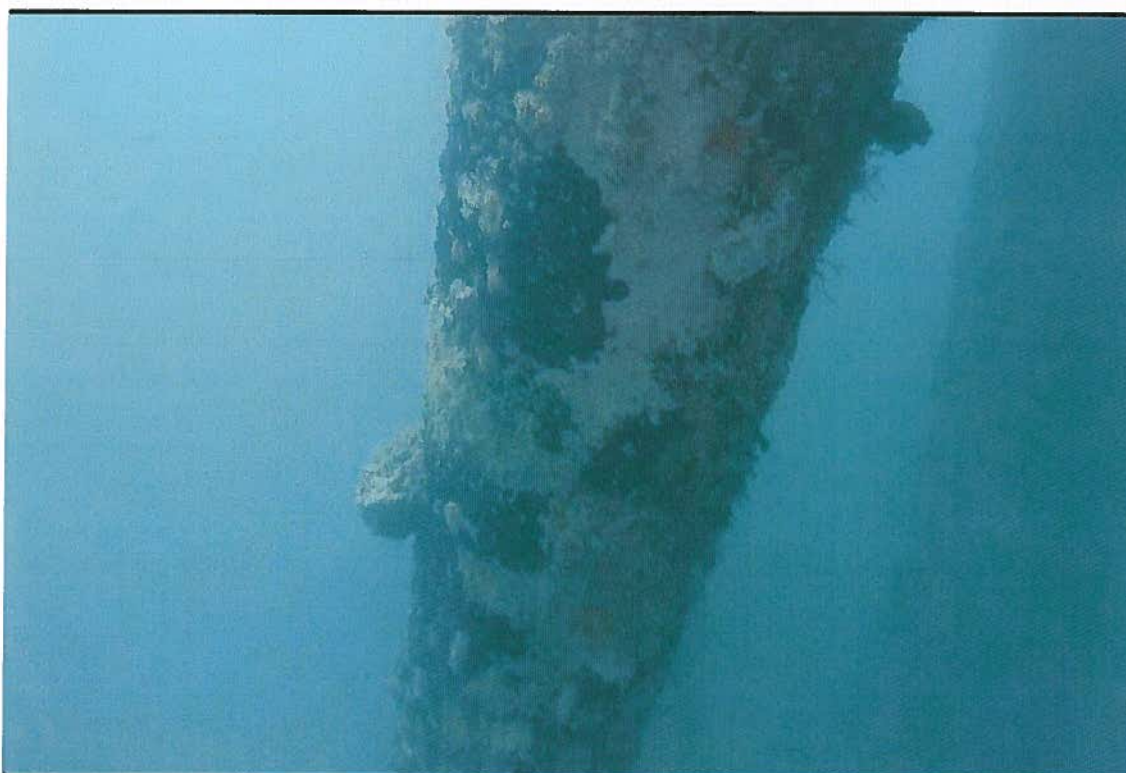
F-1 Dock Piles
