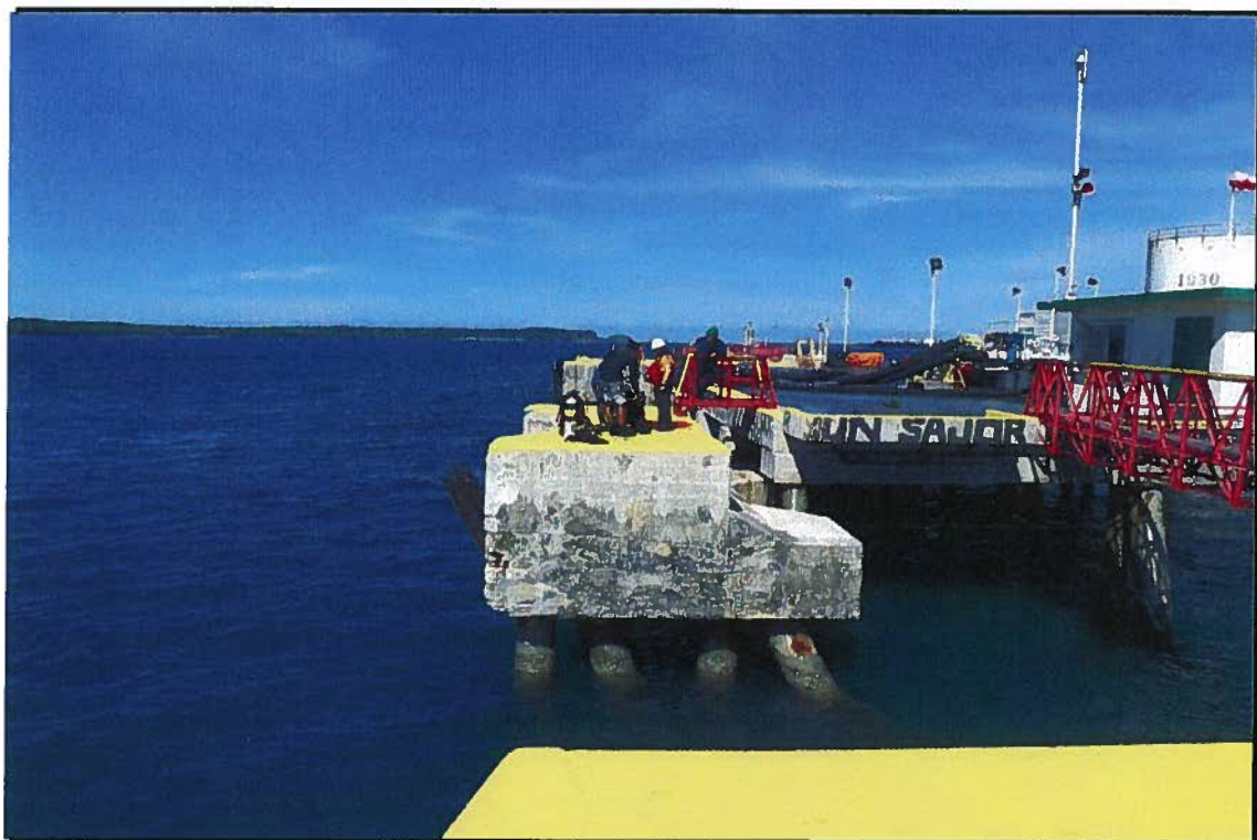
Dive Preparation for F-1 Dock Underwater Inspection
