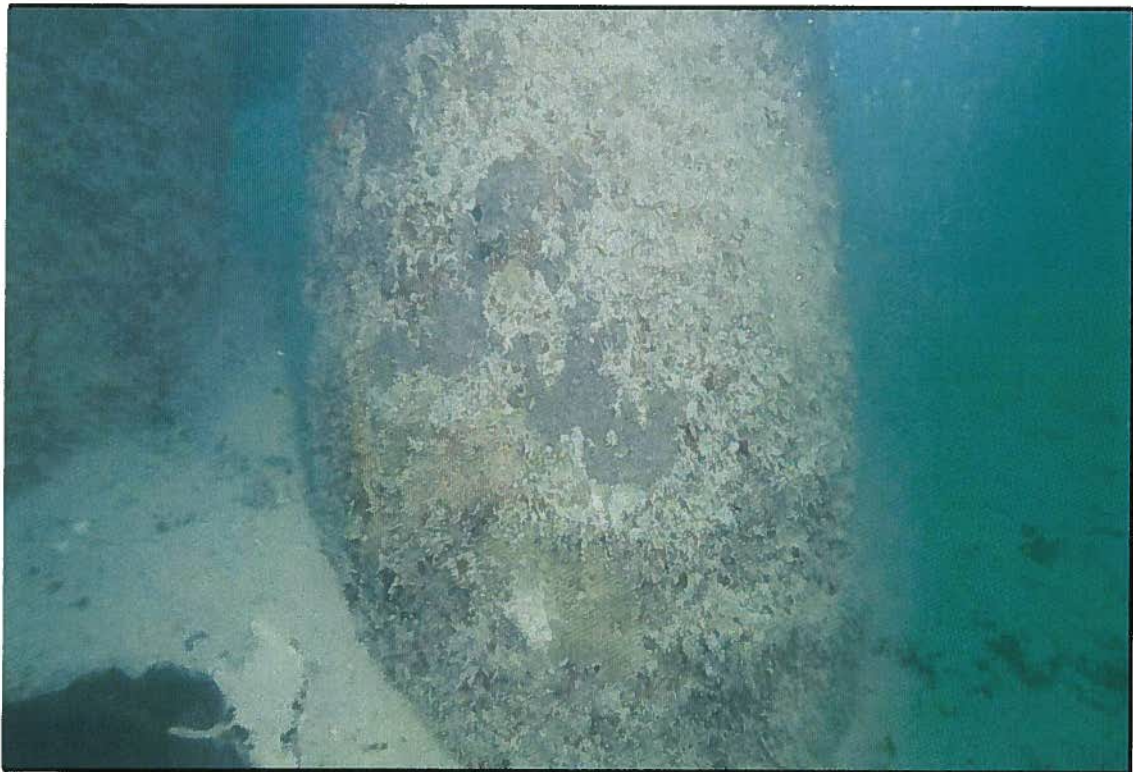
F-1 Dock Piles
