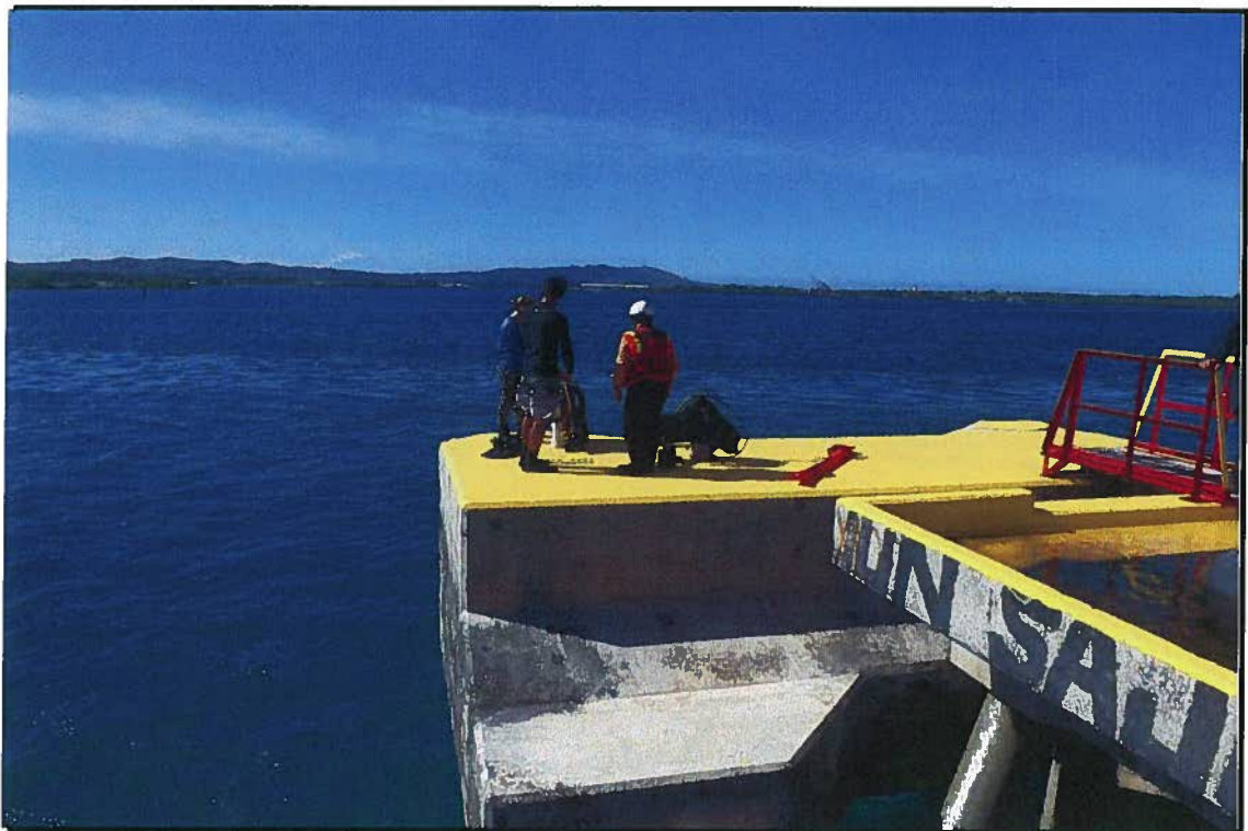
Dive Preparation for F-1 Dock Underwater Inspection
