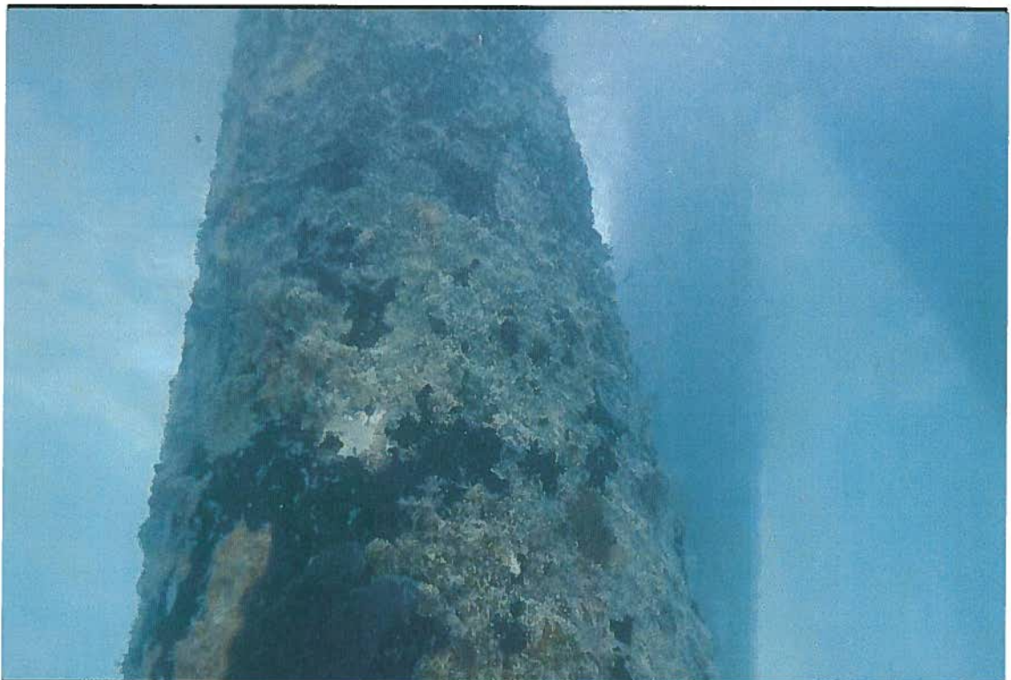
F-1 Dock Piles
