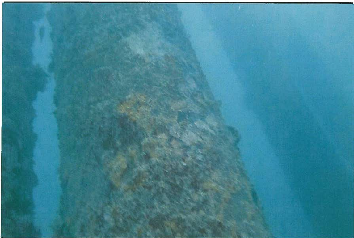
F-1 Dock Piles
