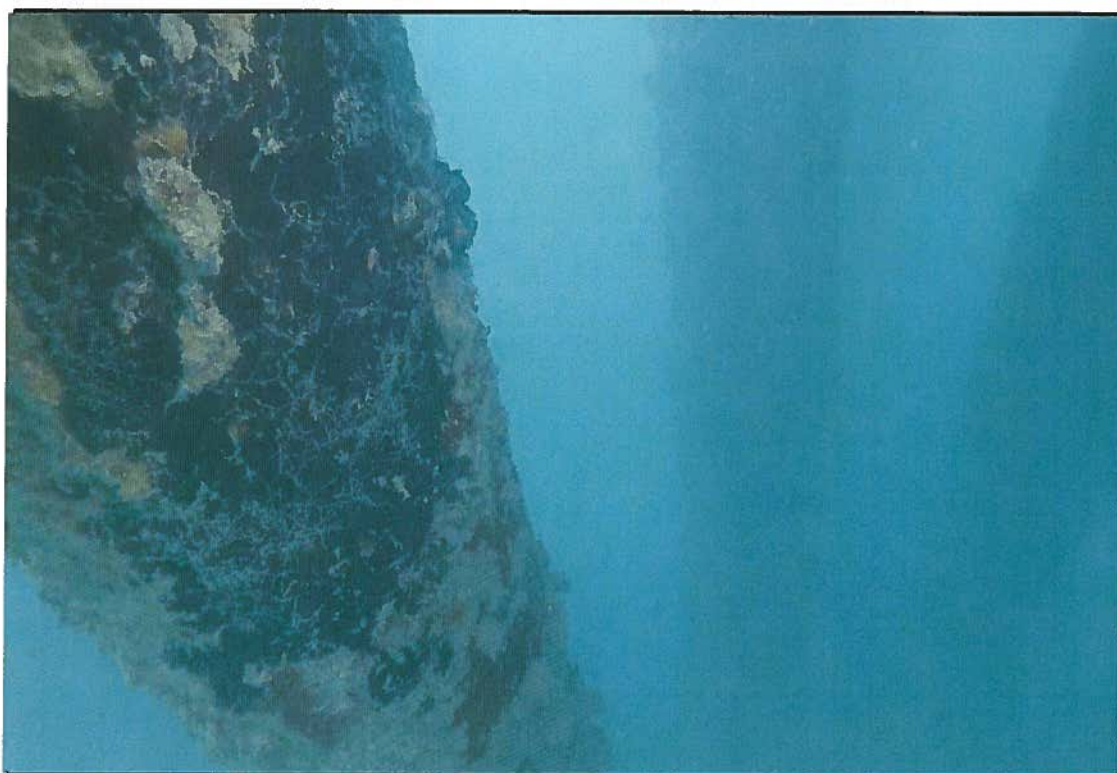
F-1 Dock Piles
