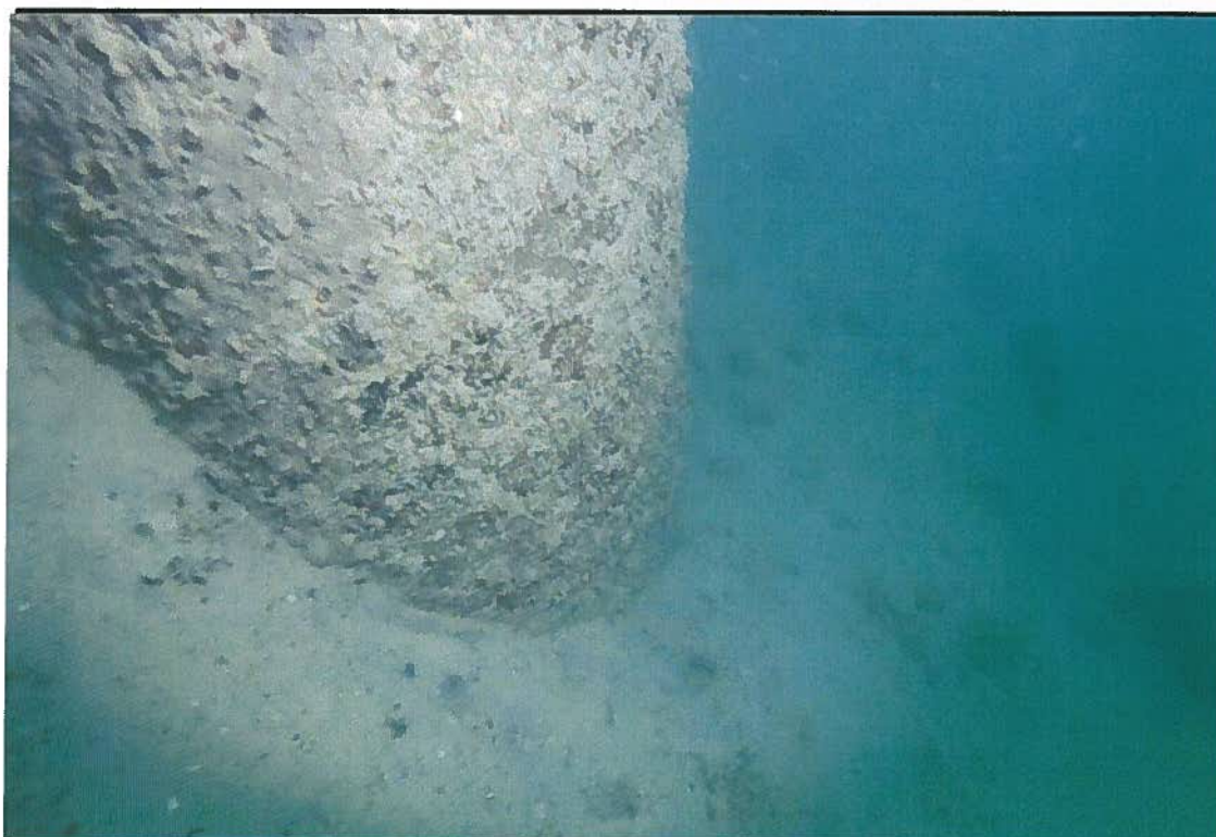
F-1 Dock Piles
