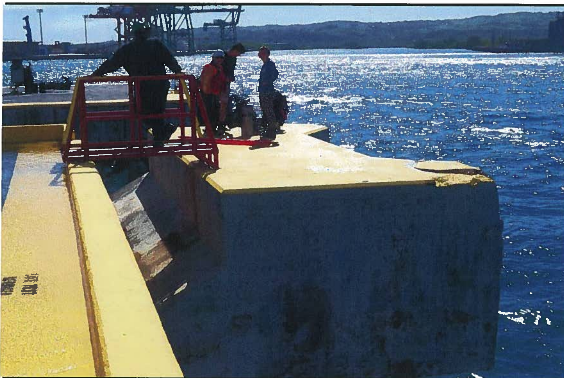
Dive Preparation for F-1 Dock Underwater Inspection
