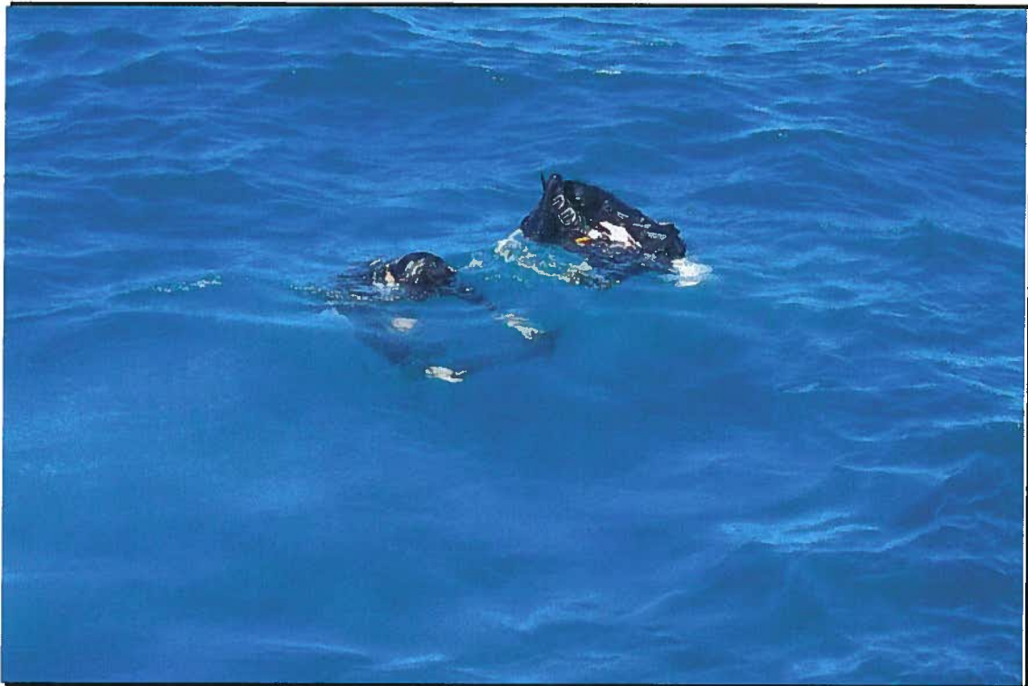
F-1 Dock Underwater Inspection Divers
