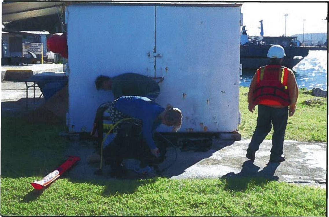
Dive Preparation for F-1 Dock Underwater Inspection
