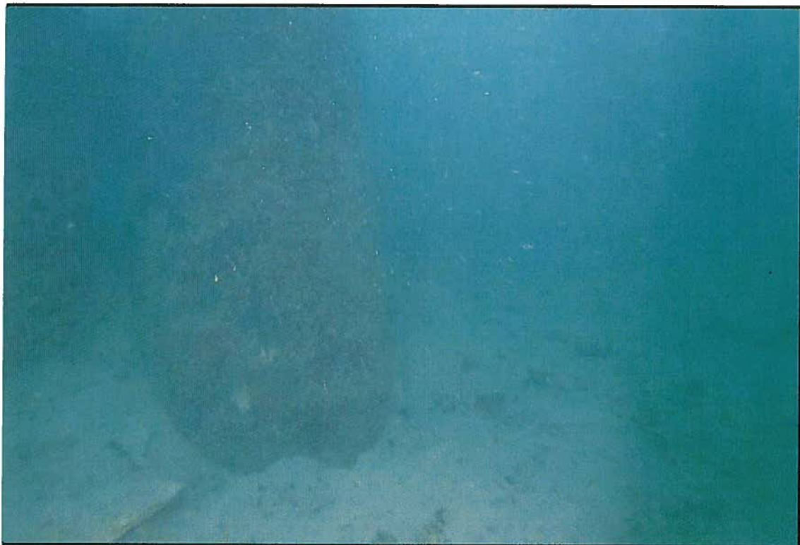
F-1 Dock Piles
