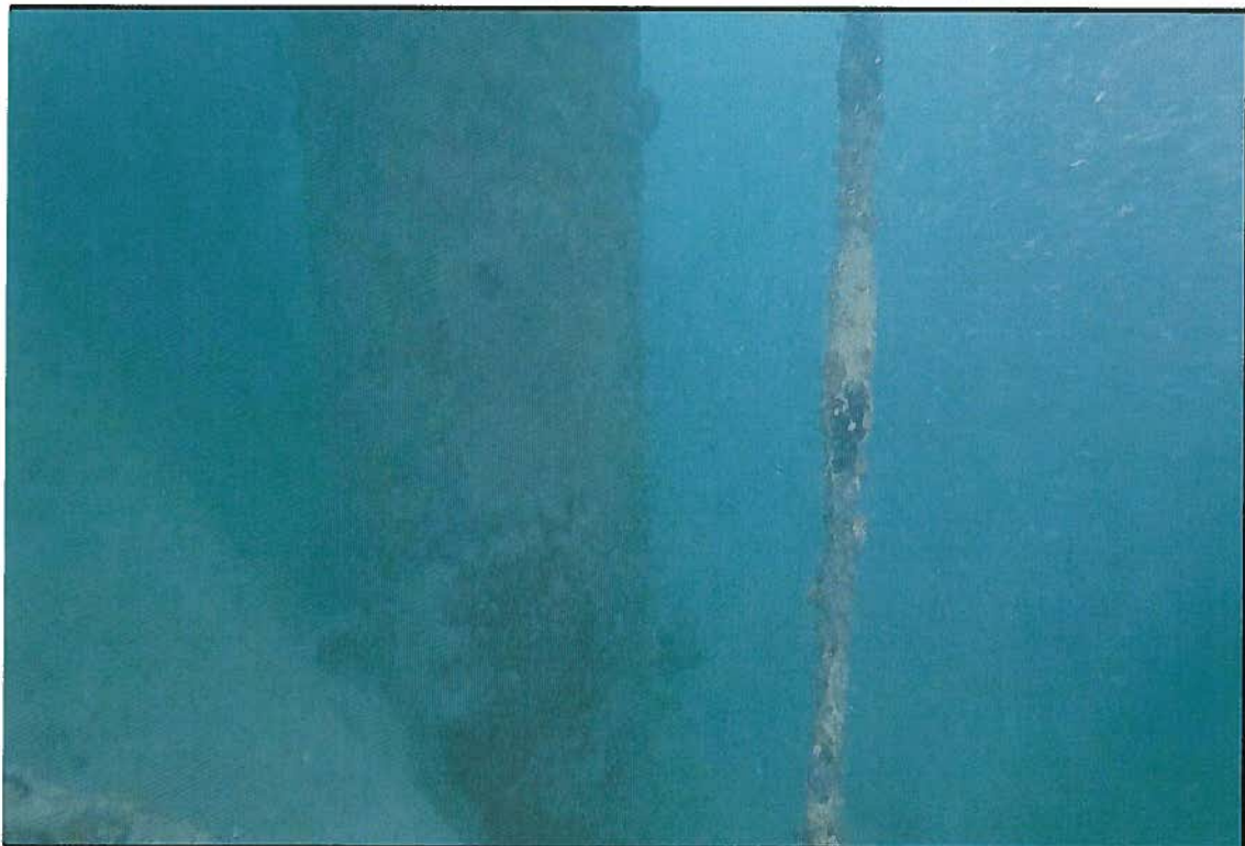
F-1 Dock Piles
