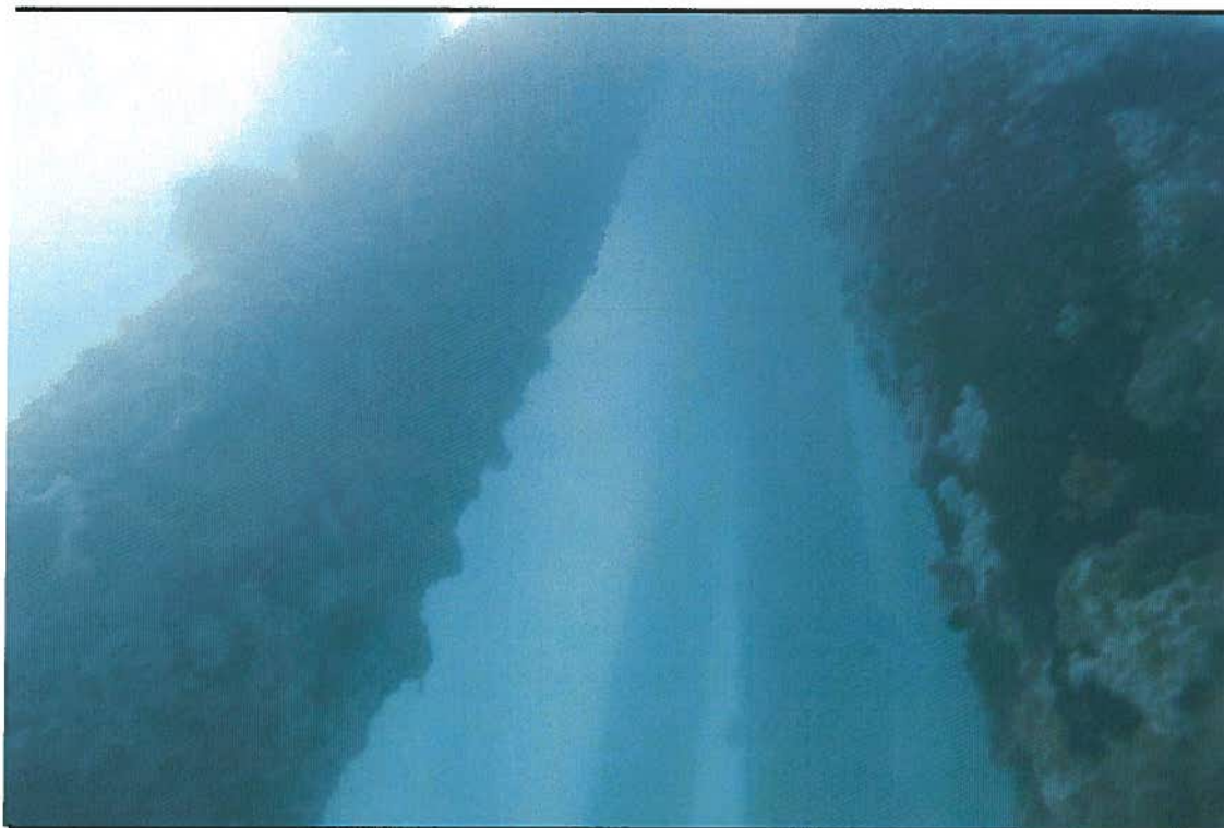
F-1 Dock Piles
