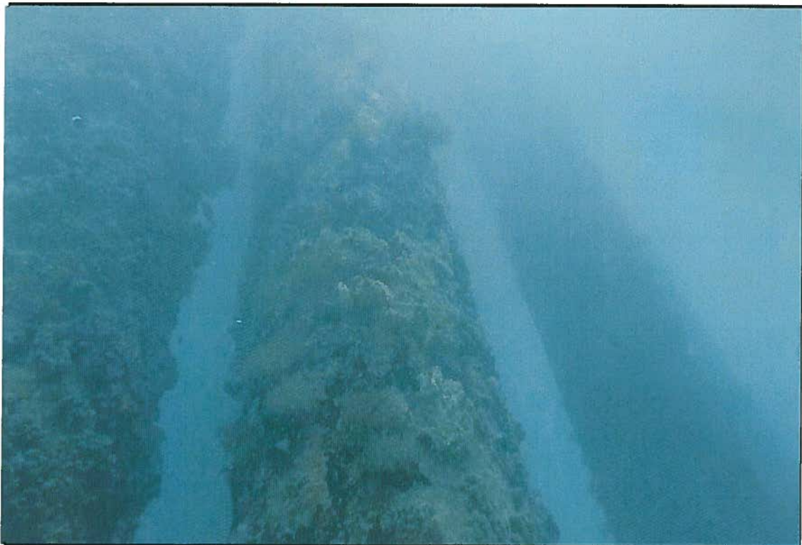
F-1 Dock Piles
