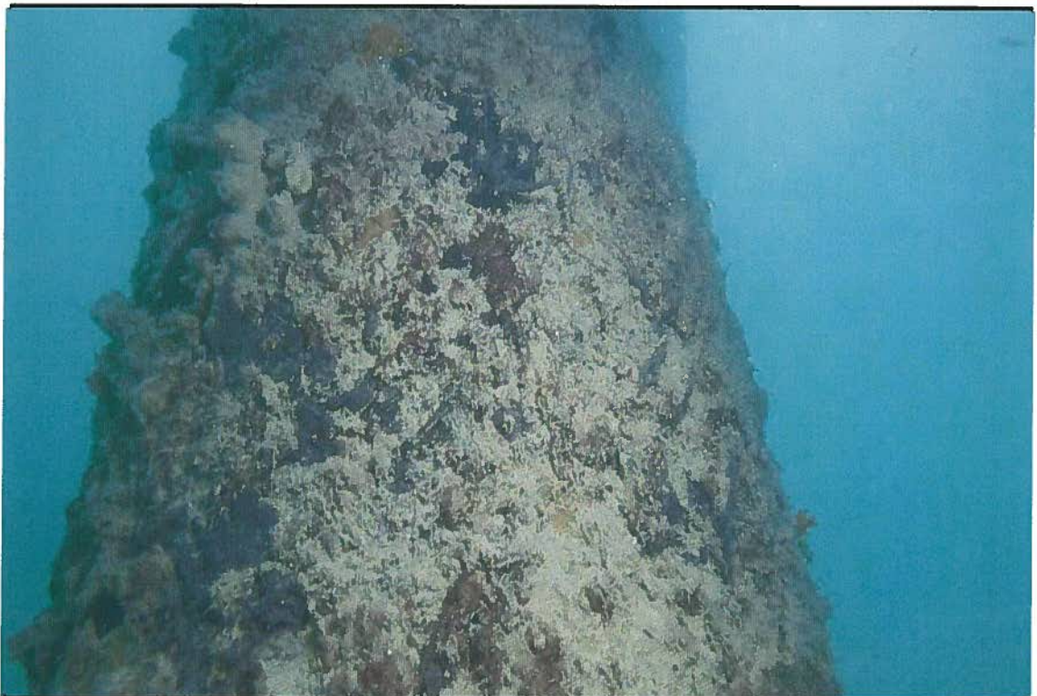
F-1 Dock Piles
