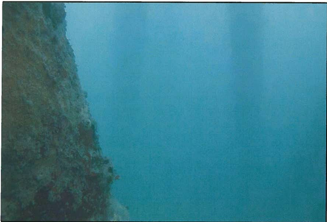
F-1 Dock Piles
