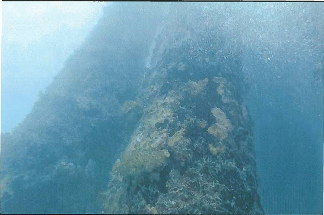
F-1 Dock Piles
