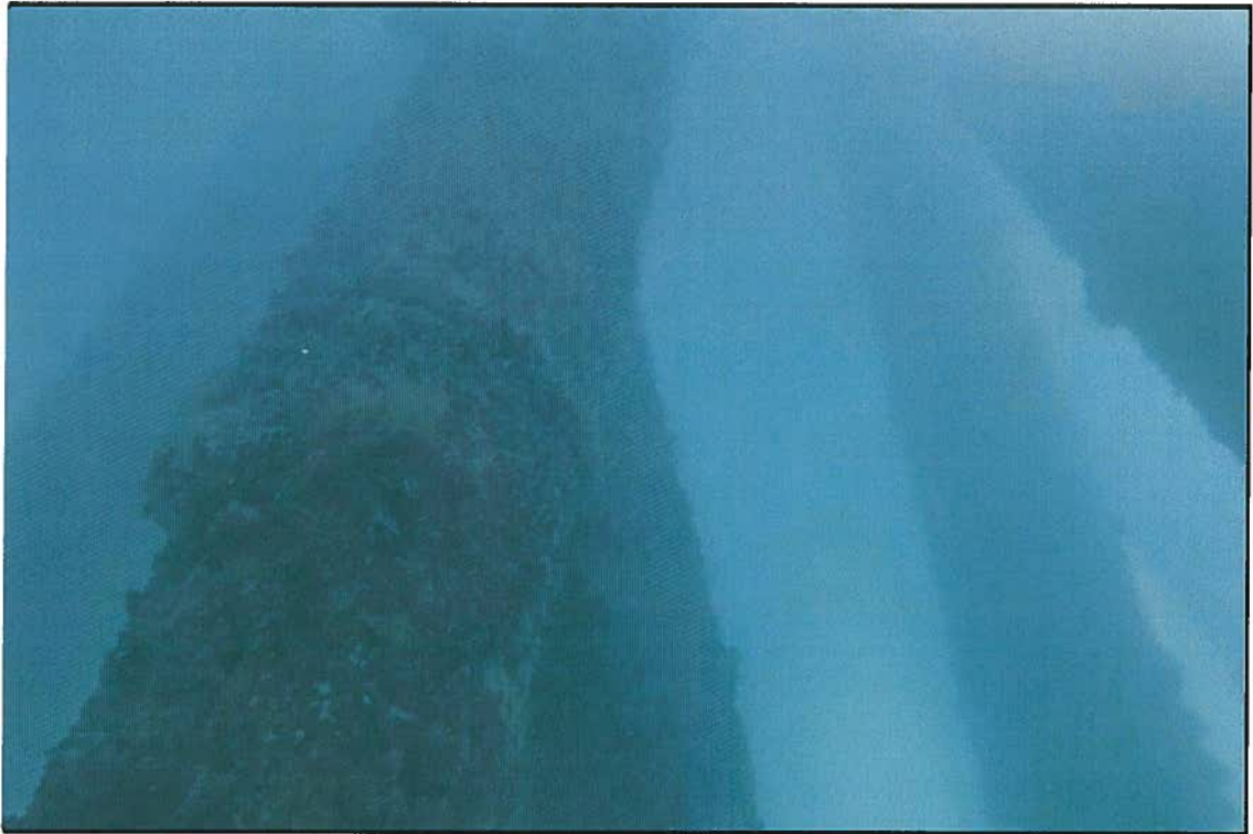
F-1 Dock Piles
