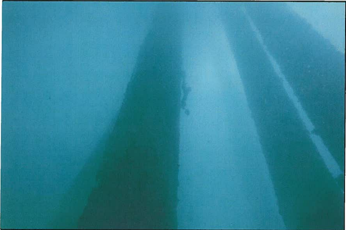
F-1 Dock Piles
