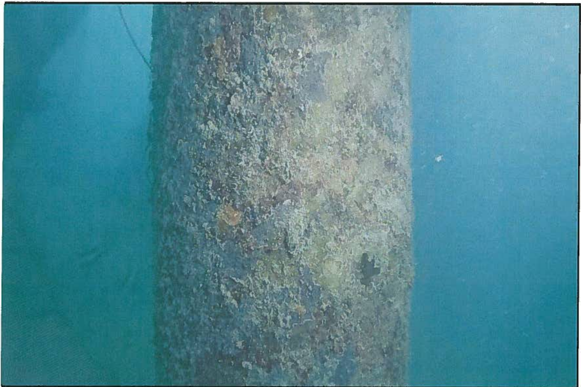
F-1 Dock Piles
