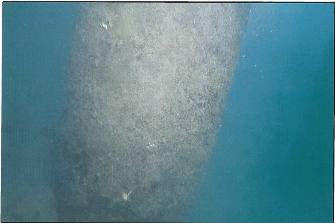
F-1 Dock Piles
