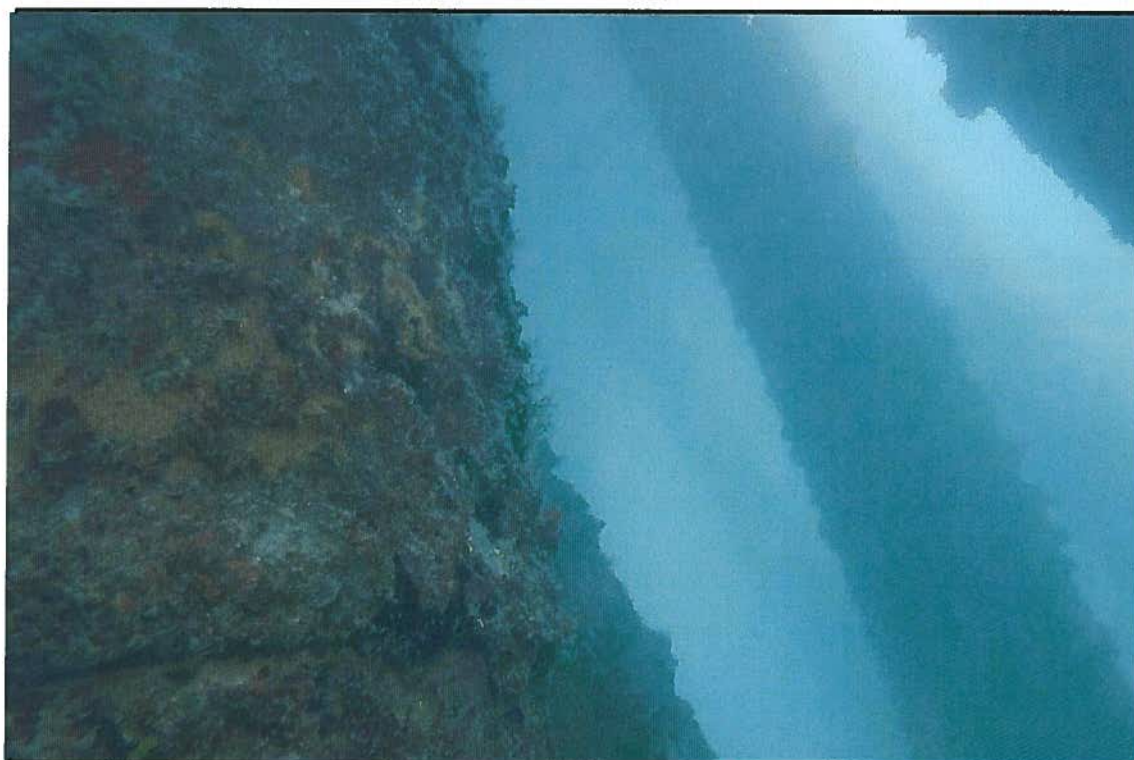
F-1 Dock Piles
