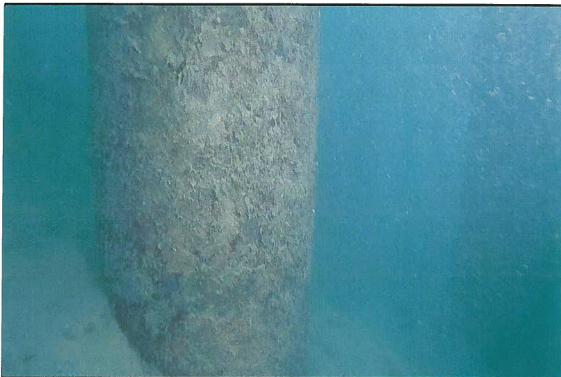
F-1 Dock Piles
