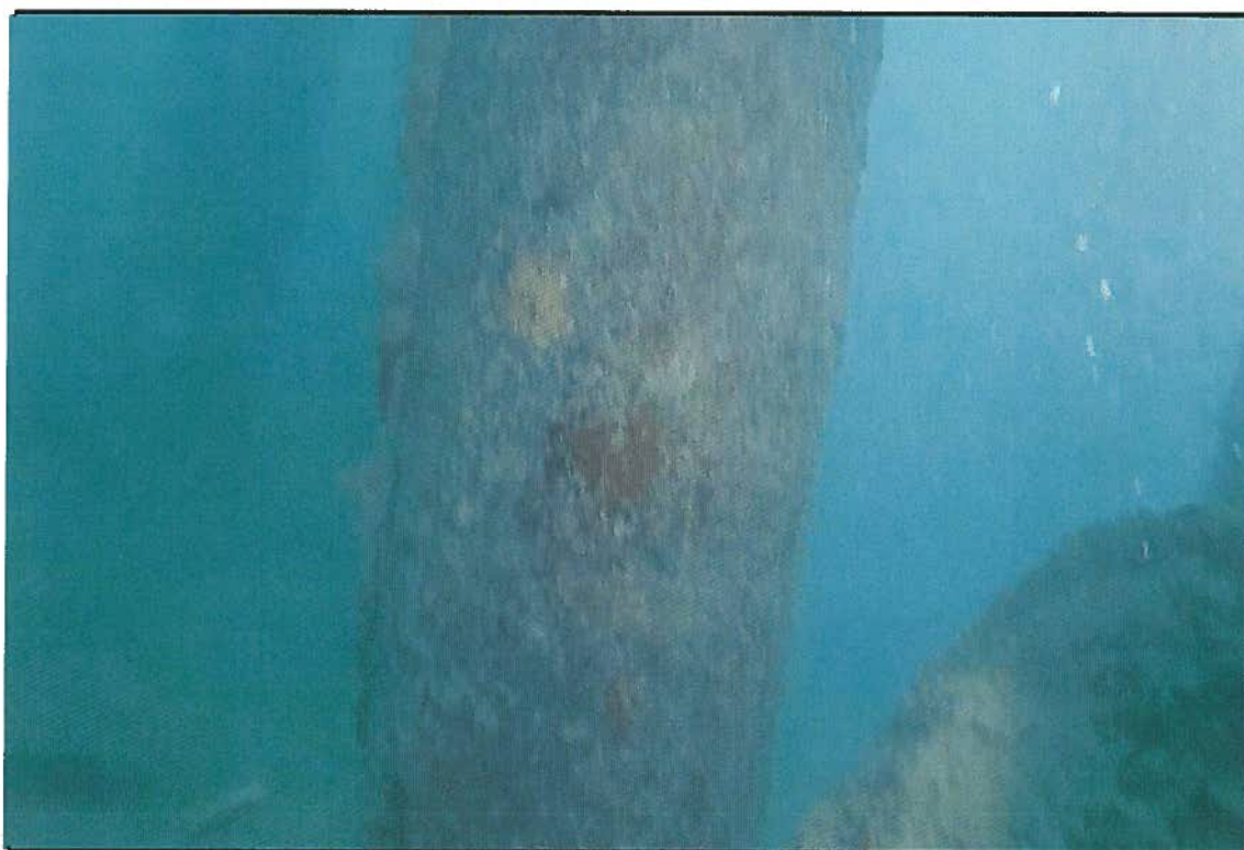
F-1 Dock Piles
