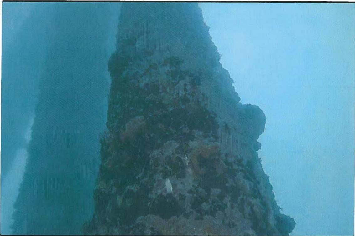
F-1 Dock Piles
