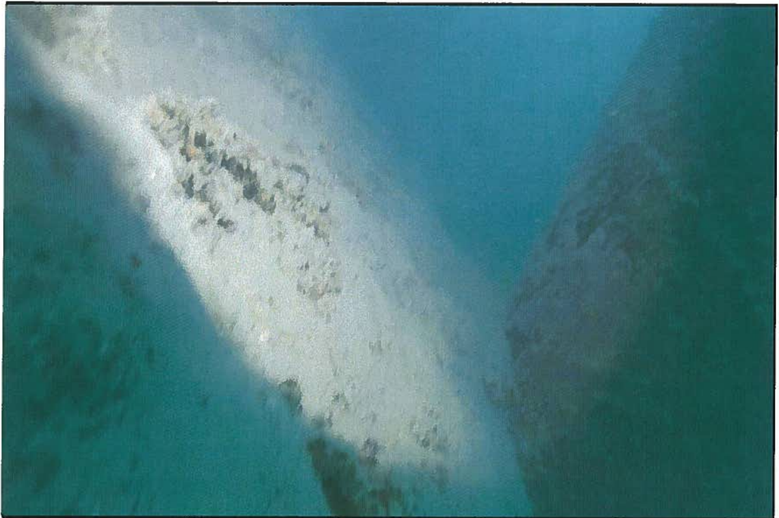
F-1 Dock Piles
