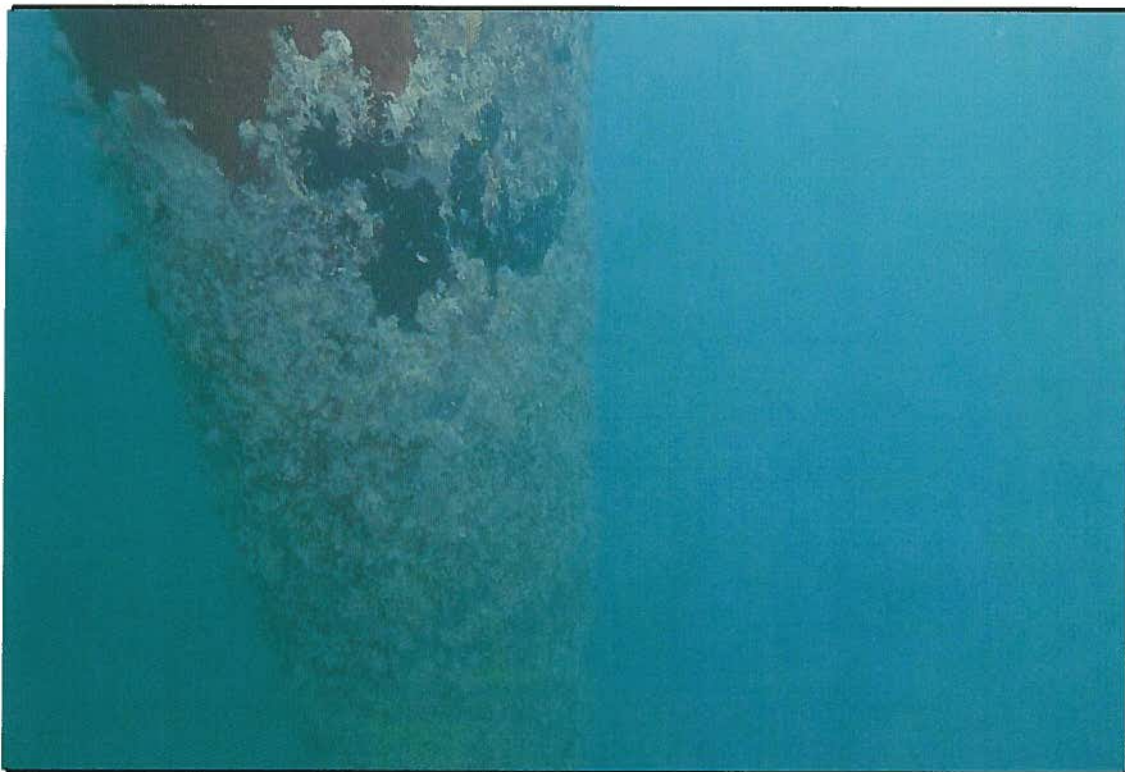
F-1 Dock Piles
