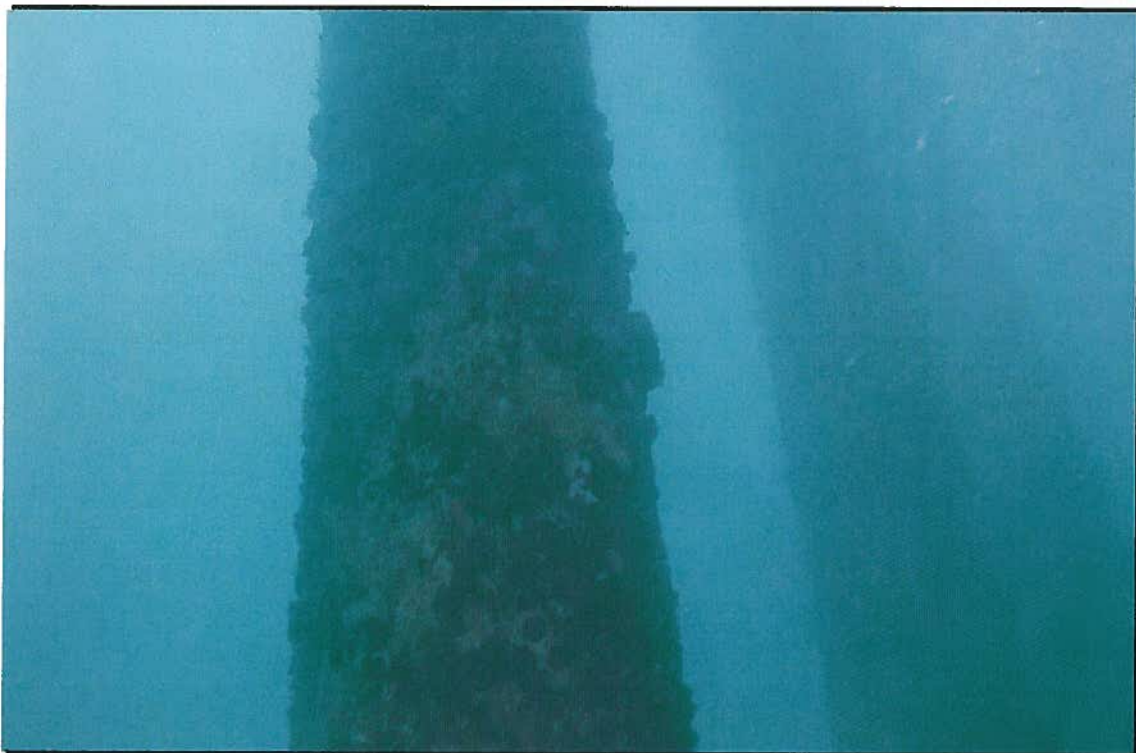
F-1 Dock Piles
