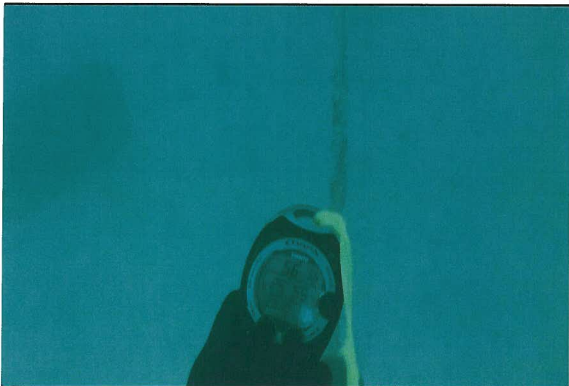
F-1 Dock Piles
