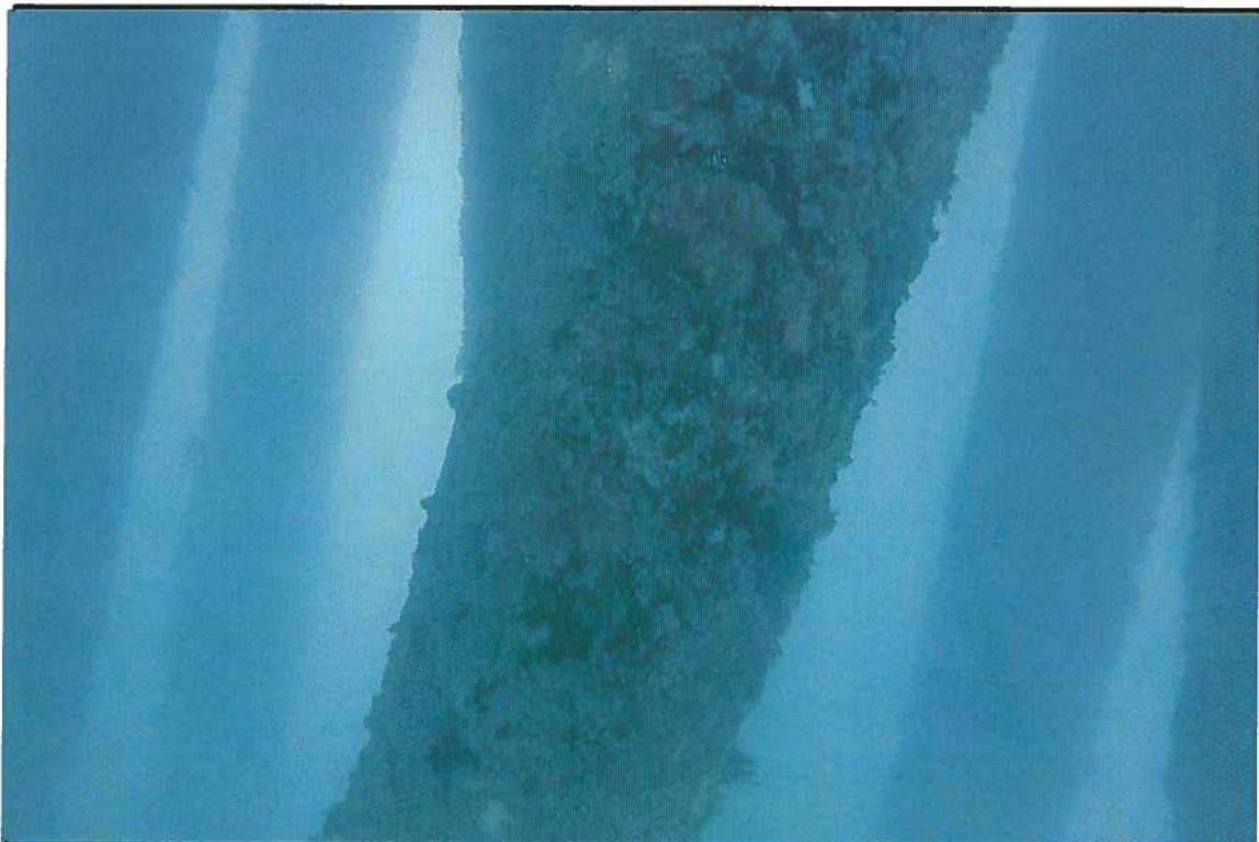
F-1 Dock Piles
