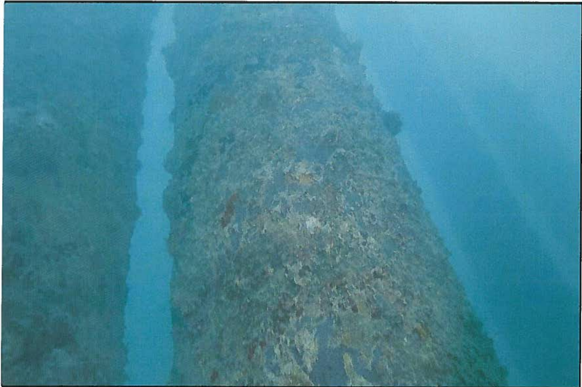
F-1 Dock Piles
