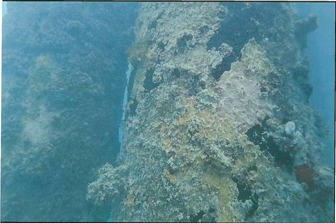
F-1 Dock Piles
