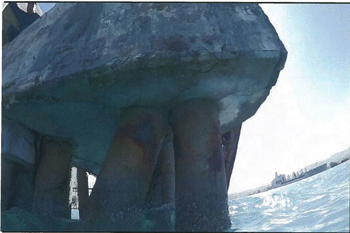
F-1 Dock Piles & Concrete Cap
