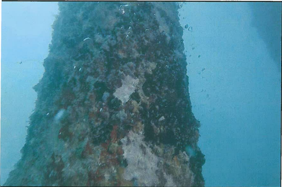
F-1 Dock Piles
