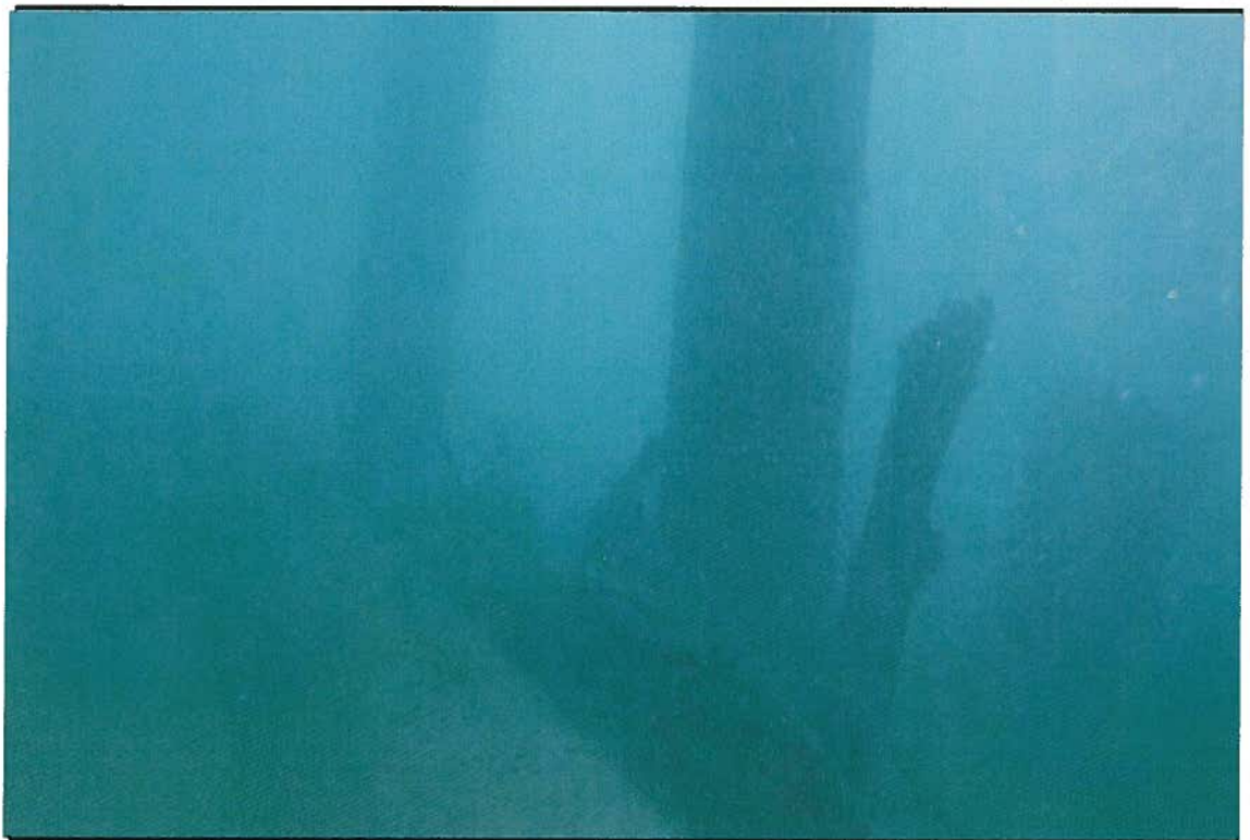
F-1 Dock Piles
