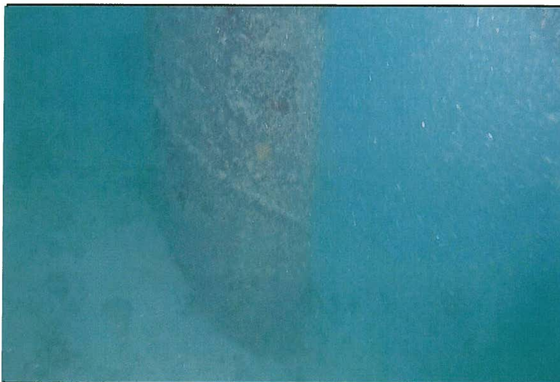
F-1 Dock Piles
