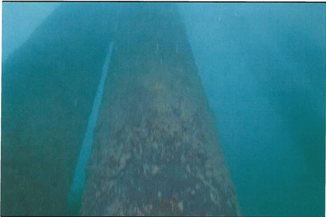
F-1 Dock Piles
