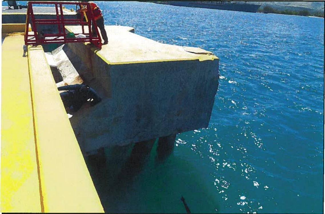
Surface inspection of Pipe Piles at F-1 Dock Fender
