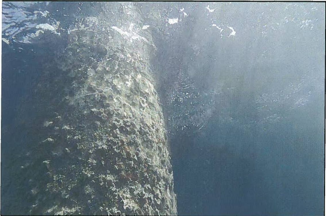
F-1 Dock Piles
