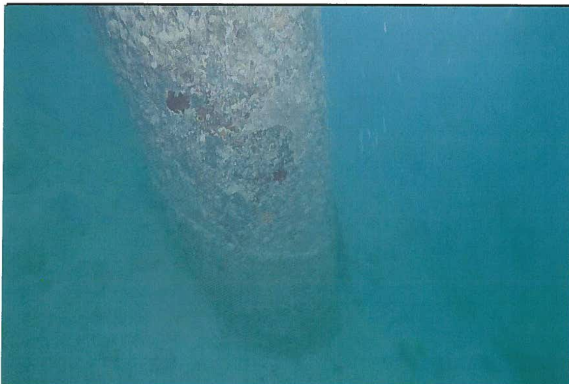
F-1 Dock Piles
