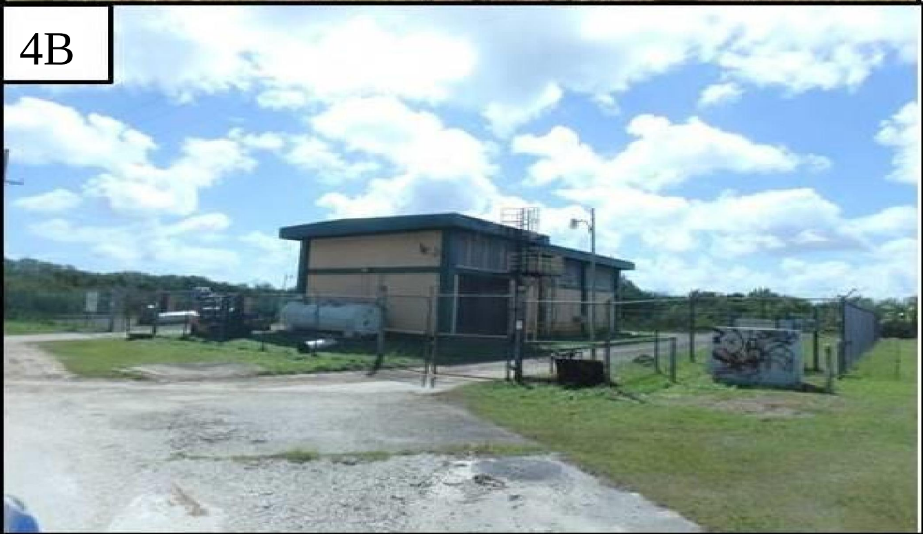
4A: Representative Easement Corridor vegetation 4B: Southern Link Pump Station
