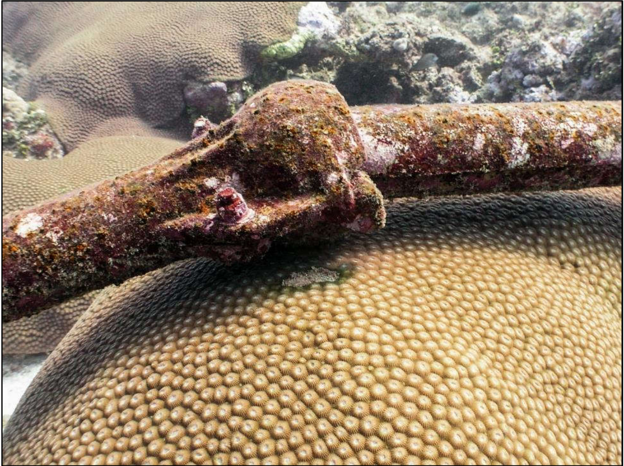
Figure 41. The ATISA Cable resting on the surface of a large Diploastrea heliopora colony. The small area of dead tissue may be an area of the colony where the cable had previously rested.
