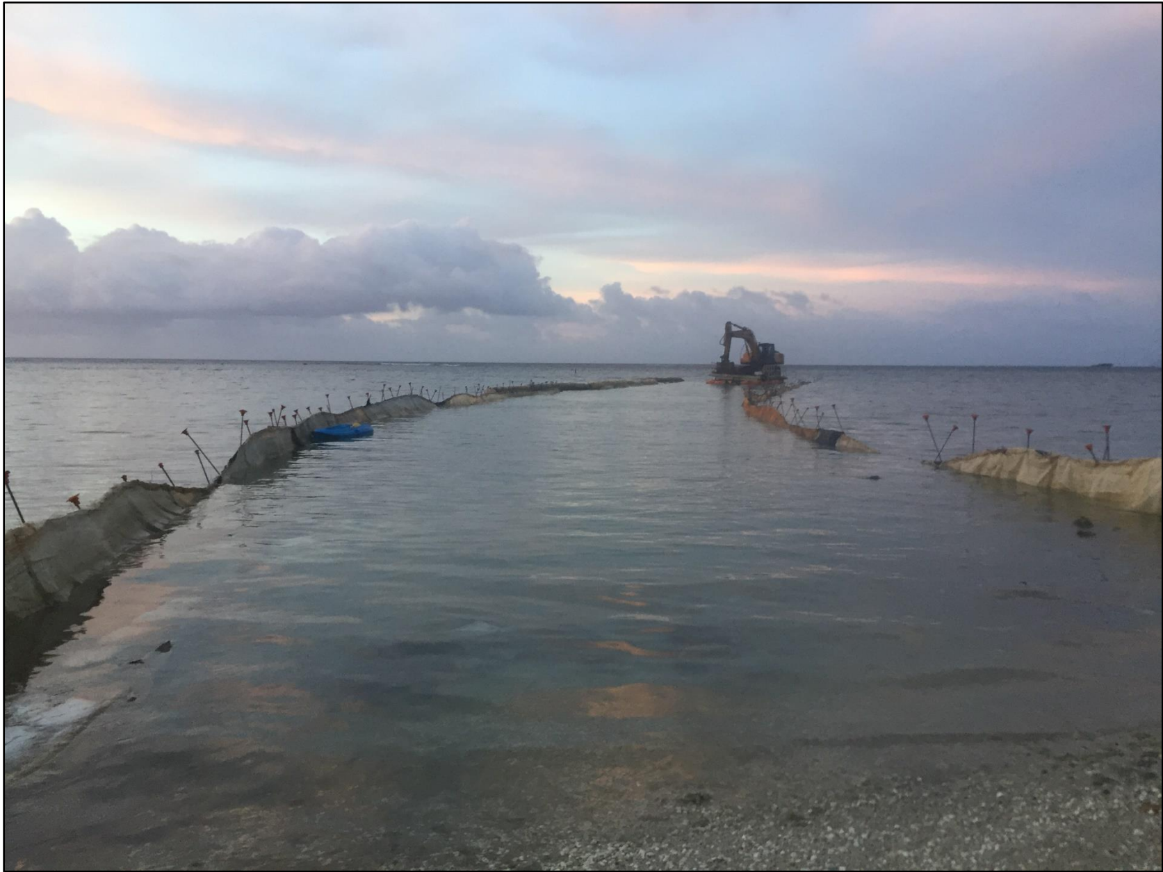
Photo 3. GTA conduit raceway construction corridor. The entrance corridor to allow for small support vessels and pedestrian access would be located entirely within this corridor and would have a smaller area.
