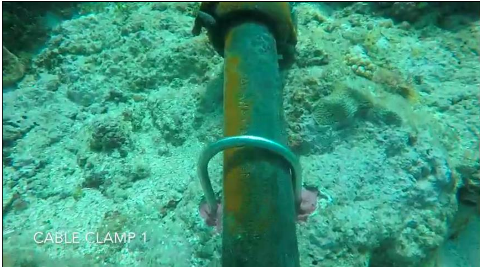
Photo 4. Cable pin installed on the ATISA Cable in 2017. The same hardware and methods would be used for the HK-G Cable pin installation.
