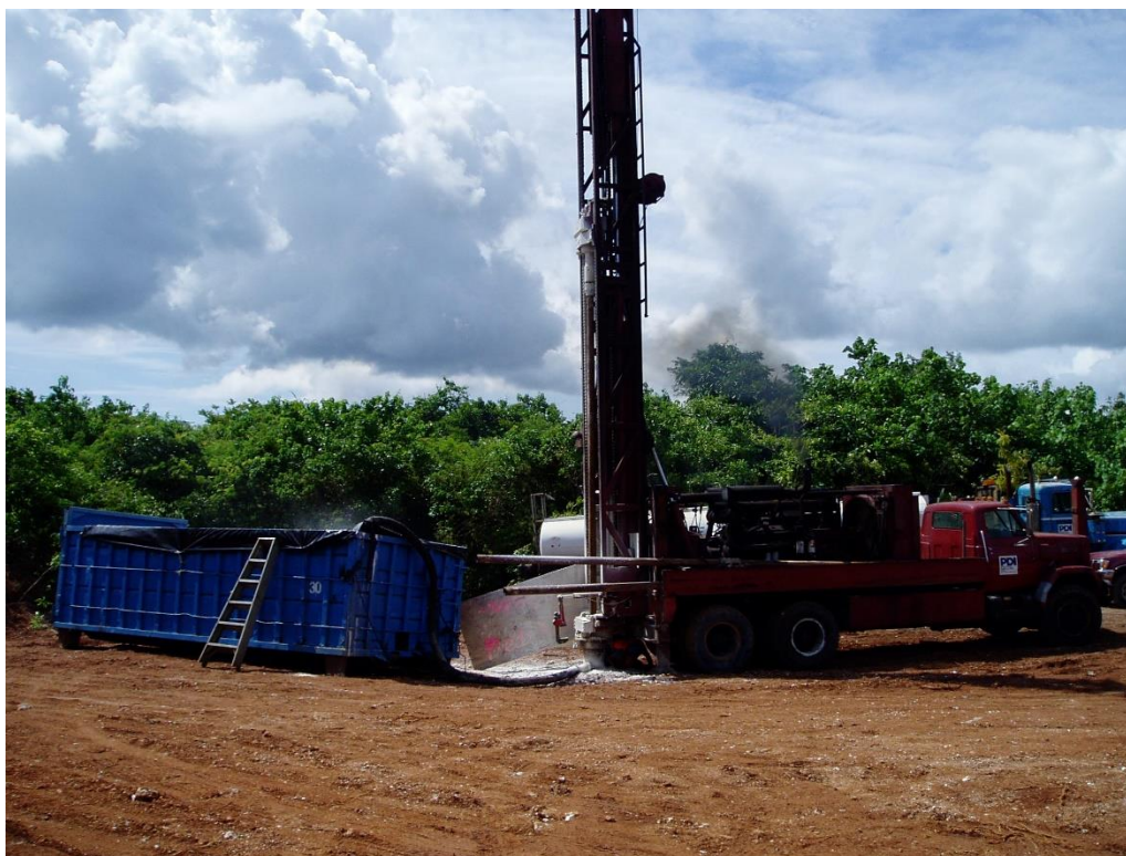
Photo 1. Typical Drill Site Layout with Air Rotary Drill Completing Deep Well
