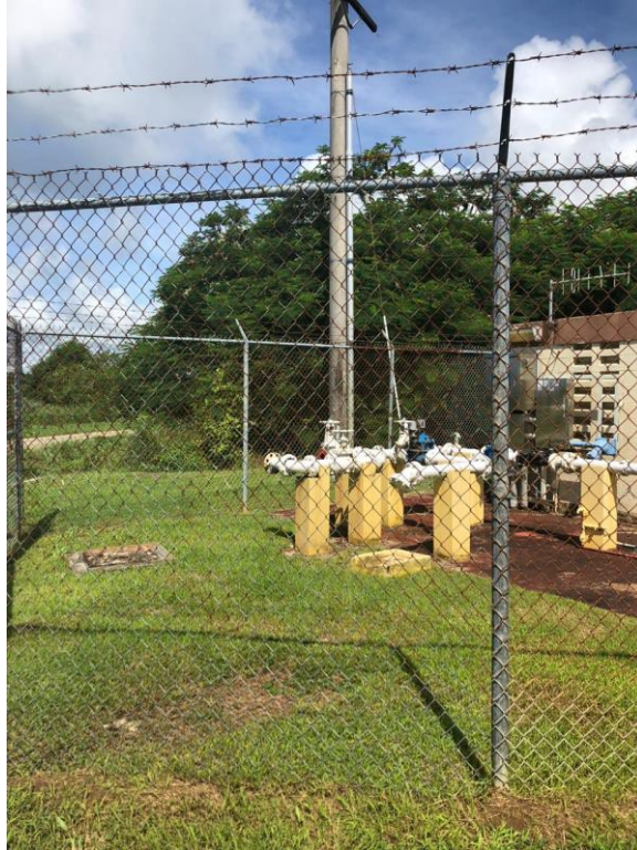
Site overview of NCS-3A
