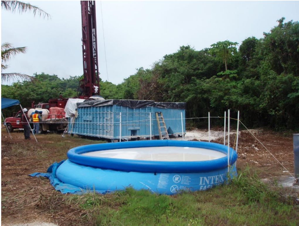
Photo 2. Typical Drill Site Layout Showing Drill Cuttings and Liquid Containment
