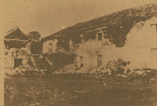
Mayulang estroktura ginen i linao gi 1902 na sakkan. 1902 Earthquake damaged building.
