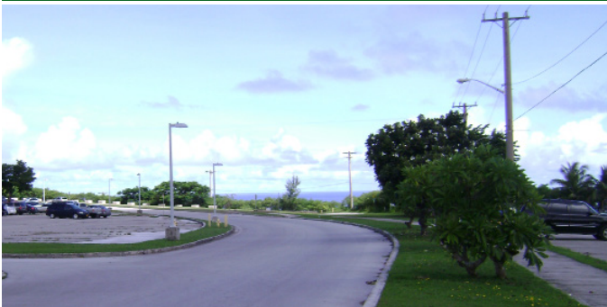
Overhead utility lines disrupt the ocean view.
