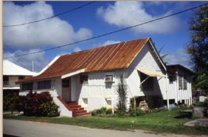
Mariano Leon Guerrero House before restoration
