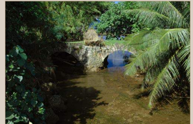
Taleyfac Spanish Bridge
