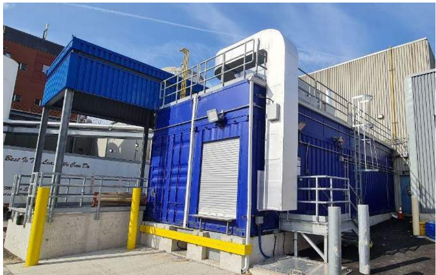
Figure 16: External View of 40' Containerized Production and Test Module with HVAC, loading dock, and utilities. (Source: Giant Containers, Labatt Brewing)
