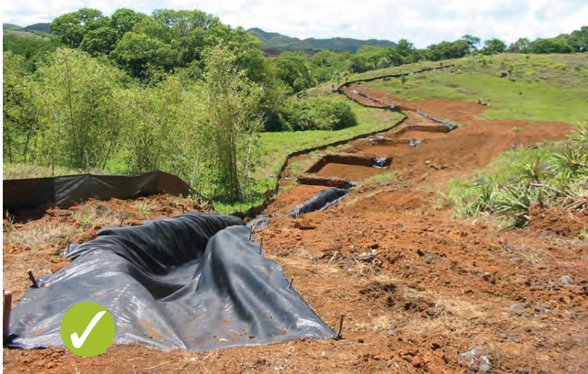
Good use of lined diversion swale to convey runoff to a series of sediment traps.
