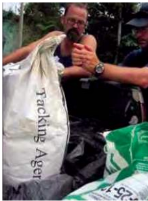
The hydroseed mix is a combination of seed, paper or wood fiber mulch, binder (tackifier) product, and sometimes fertilizer.
