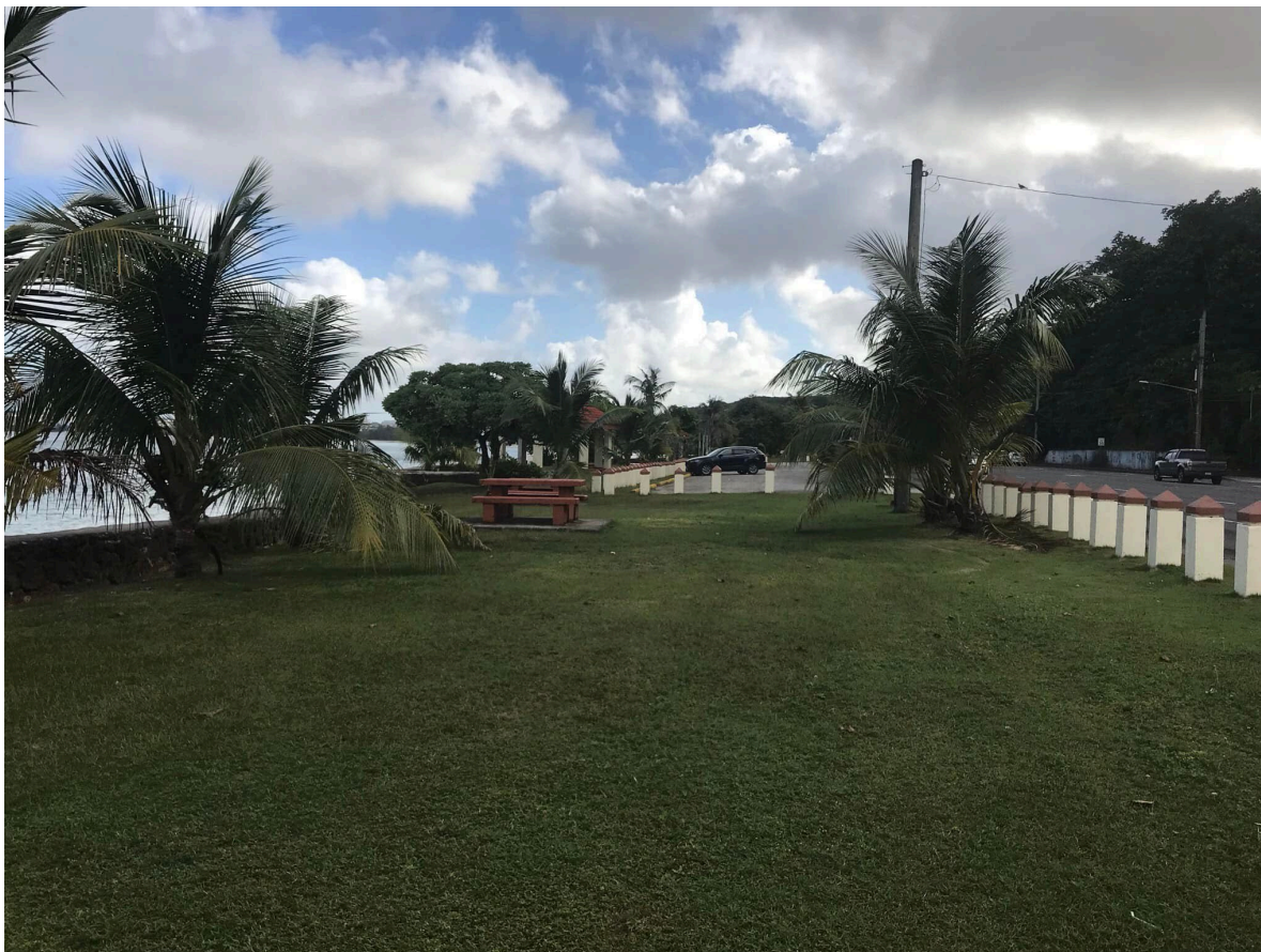
Figure 12: Relative elevation of current seawall and South Marine Corps Drive at Trinchera Beach Park. Photo by USACE staff taken on January 14, 2022.
