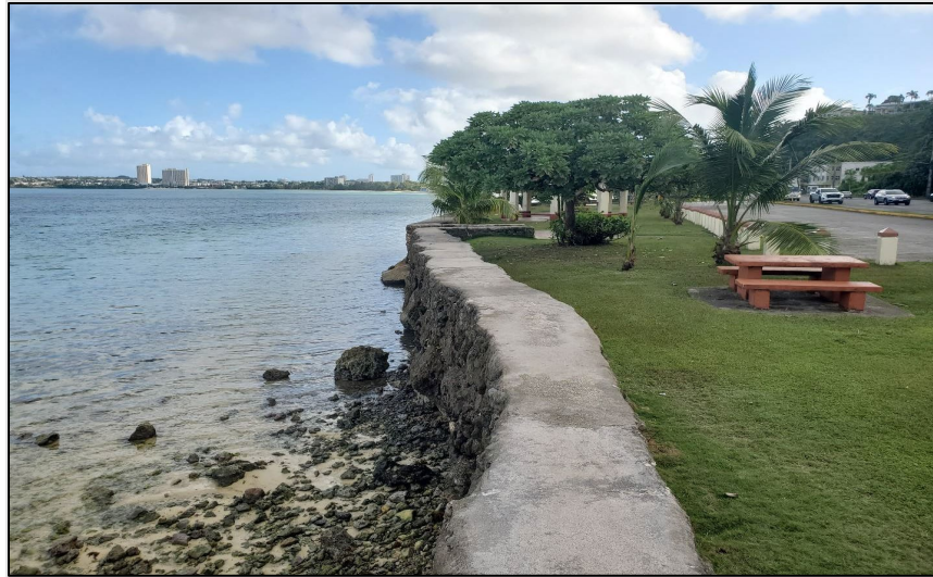
Figure 4: Existing seawall at Trinchera Beach Park, facing northeast (USACE 2022a)
