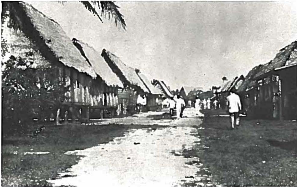
RESIDENTIAL AREA, CIRCA 1920. Constructed largely of local materials, the typical family home of this era not only lacked modern conveniences such as running water but was subject to frequent damage by the elements. Photo: Flores Memorial Library.
