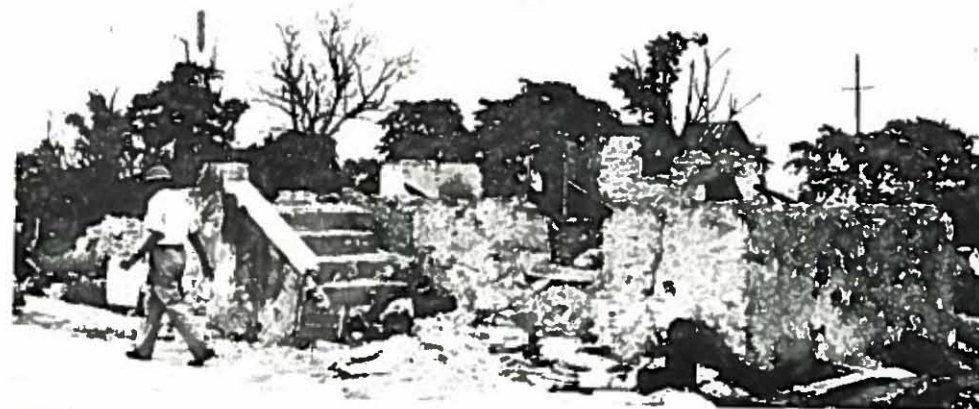
BY THE END OF WORLD WAR II, nearly all of the homes in most villages had been destroyed or heavily damaged. Photo: Flores Memorial Library.
