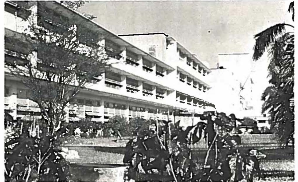
GUAM MEMORIAL HOSPITAL. This modern 236 bed reinforced concrete building has served Guam's civilian community since 1956. Due to certain design deficiencies which make it impractical to expand the present facility, studies are underway to design an entire new hospital complex.
