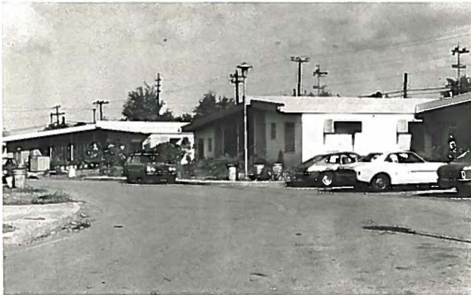
RESIDENTIAL AREA, 1973. The majority of homes constructed today are modern typhoon-proof concrete structures. Pictured above are homes provided by the Government of Guam for low-income families who are charged a nominal rental fee consistent with their means.
