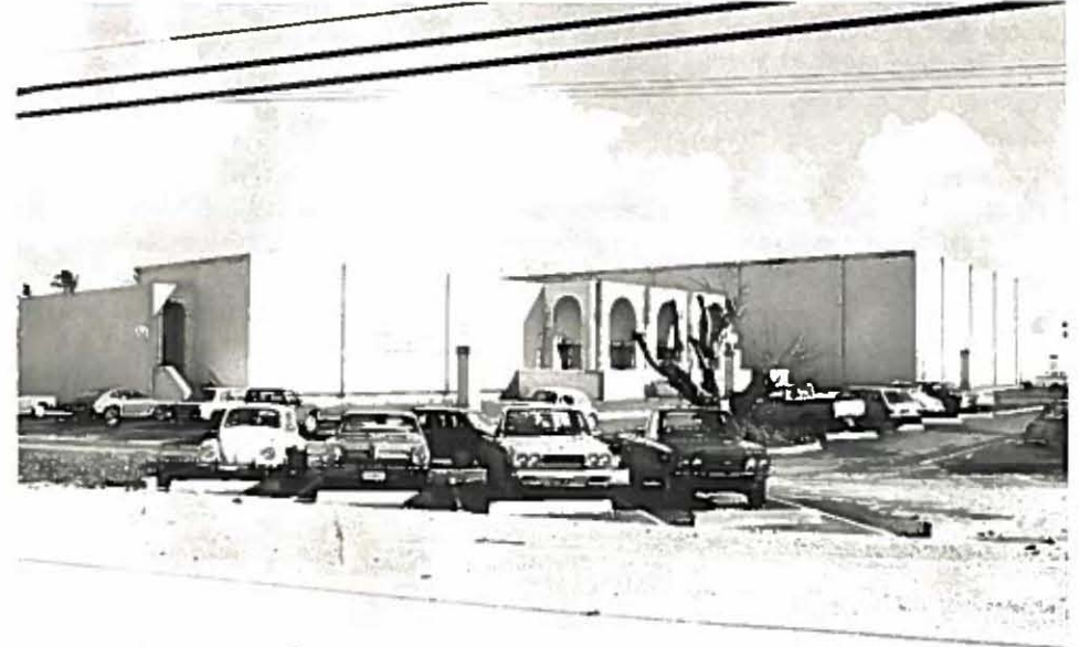
CENTRAL PUBLIC HEALTH AND SOCIAL SERVICES DIAGNOSTIC AND TREATMENT FACILITY. Dedicated in February of 1973, this building serves as the headquarters for some 300 employees charged with improving the health and well-being of island residents.
