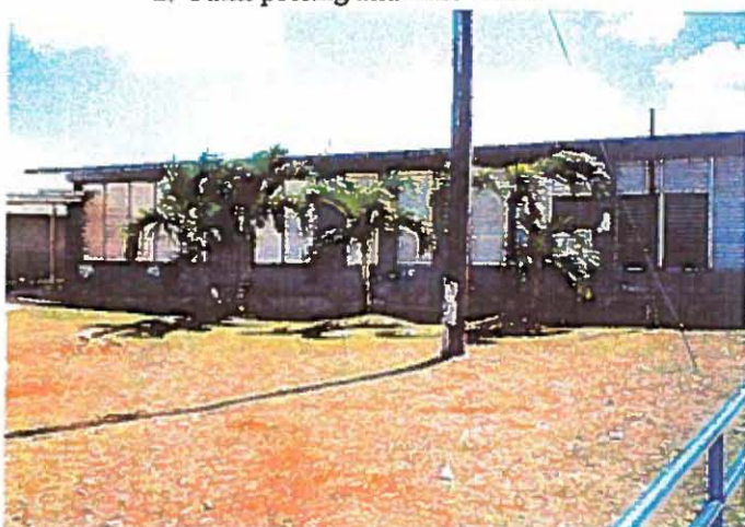
4. Exterior view of classrooms
