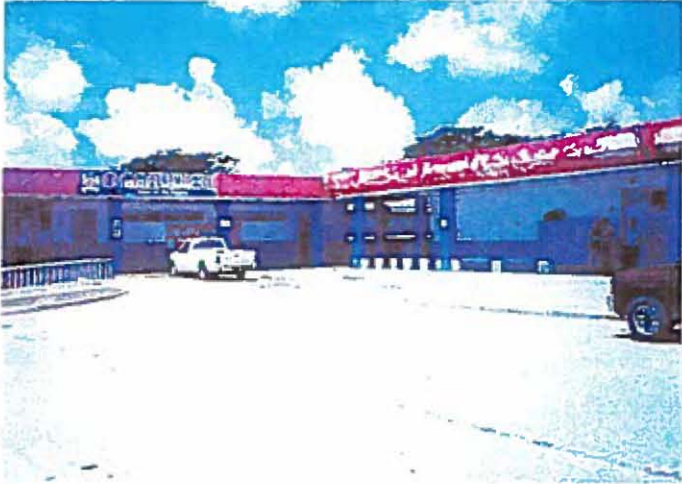
1. Entrance to the administrative building in need of new paint
