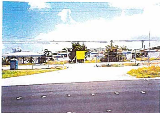
2. Removal of Paka-related debris
