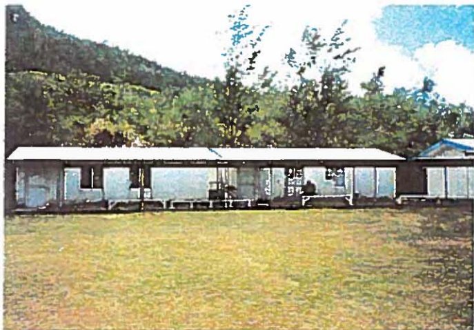
5. Exterior walls covered with algae
