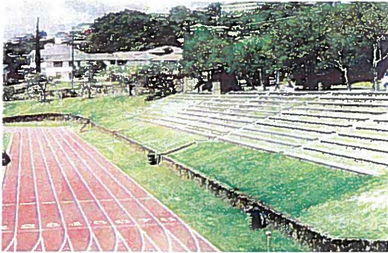
1. Treated wooden seats, set into the hillside, produce attractive yet sturdy athletic field stands.
