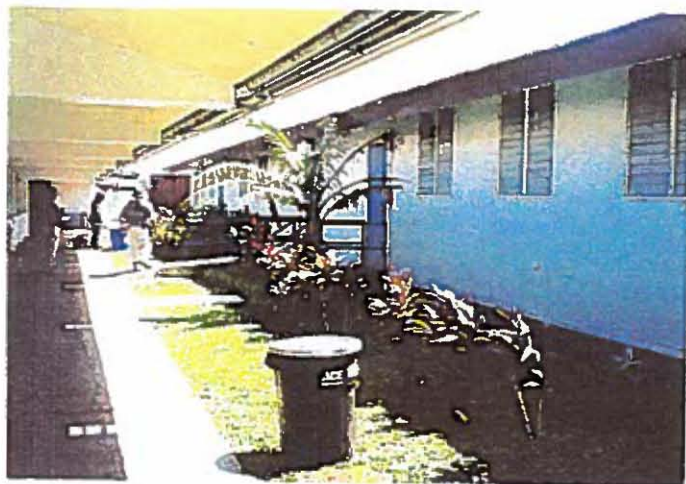
5. A permanent wing corridor adjacent to temporary classrooms
