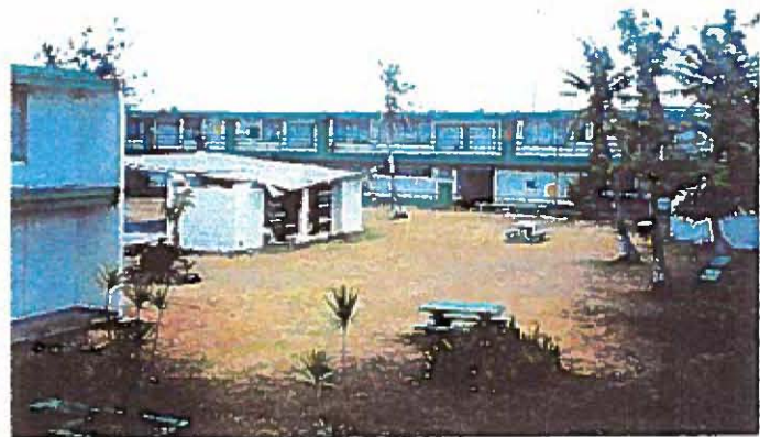
10. Courtyard with demolished stage
