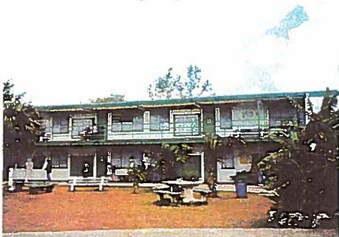
11. Concrete table with seats need new paint coat
