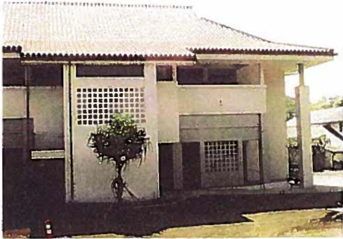
4. Building elements: Sloped tile roof, roof overhangs, and decorative wall grills.
