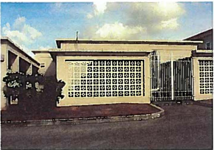
6. Screened mechanical area at Tamuning Elementary.
