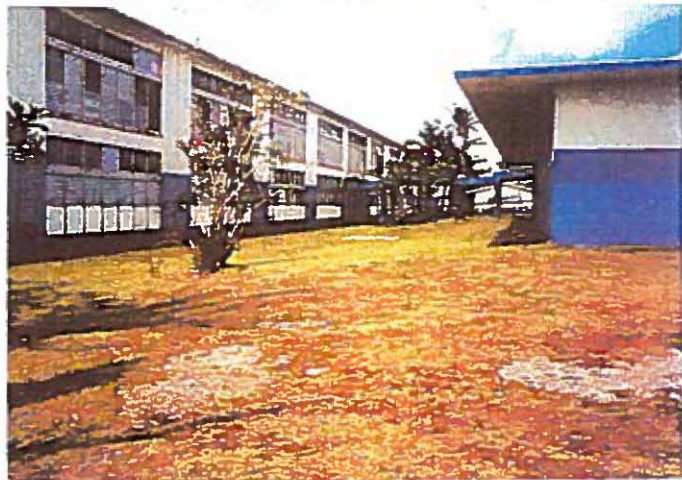
8. Exterior view of buildings
