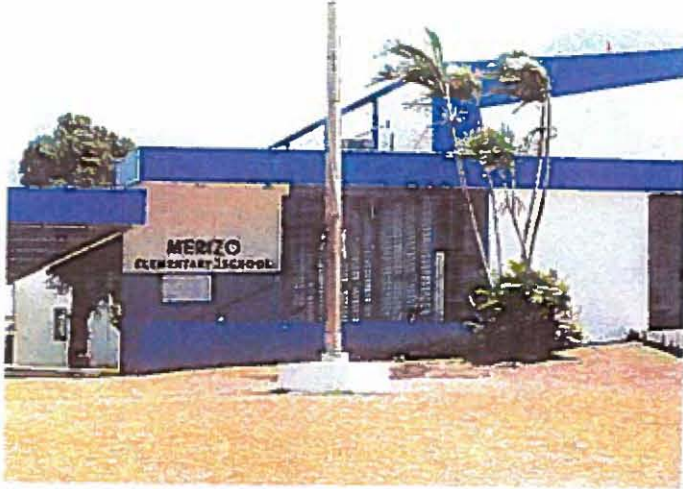
7. Exterior view of main building
