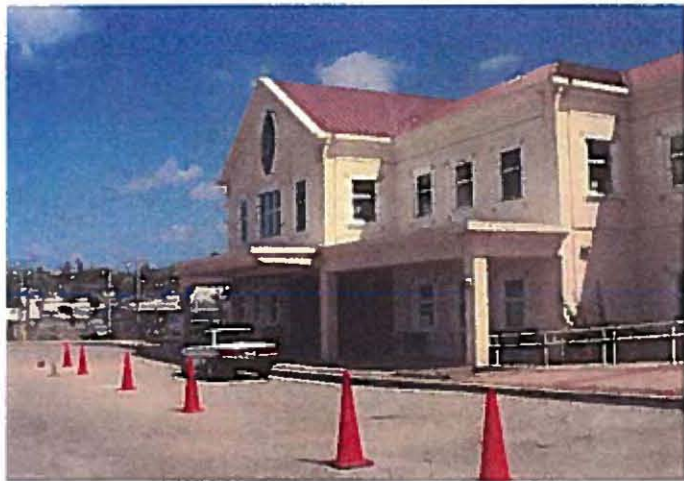
1. Tamuning Elementary front facade and drop-off area.
