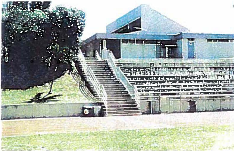
2. Concrete viewing stands are set into hillside.
