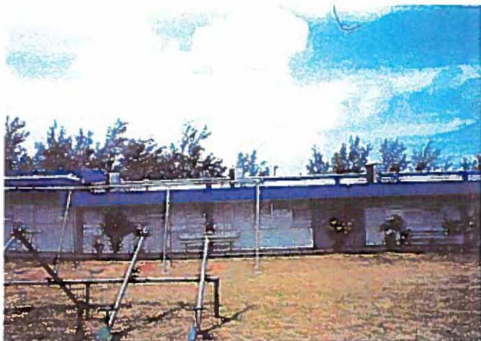
2. Exterior view of main building
