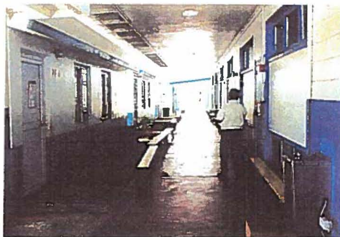
4. Hallway inside the building
