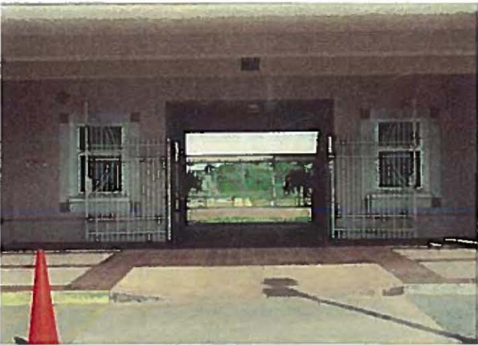
1. Courtyard building entry gate at Tamuning Elementary.
