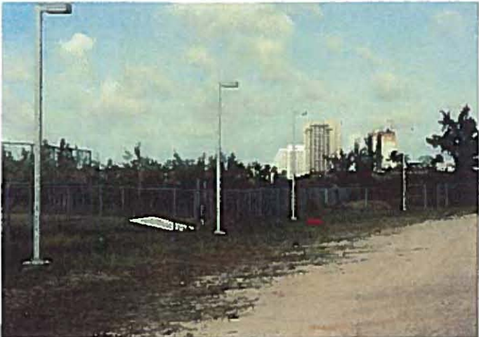
4. Security fence and lighting
