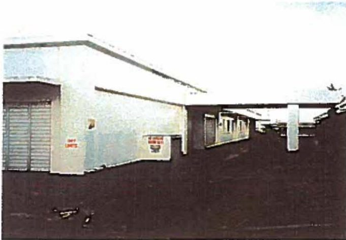
3. Permanent classrooms located west of main building
