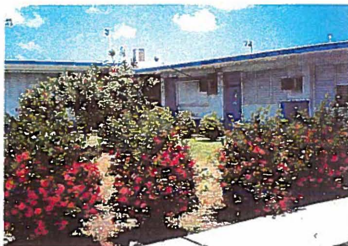
8. Shrubs along walkway
