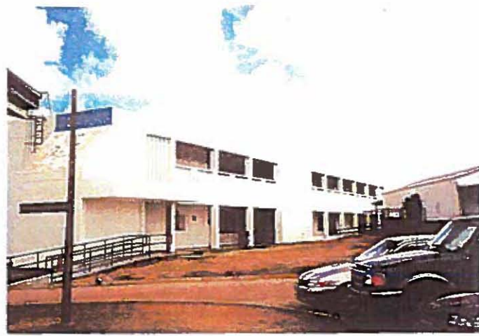
2. New building annex
