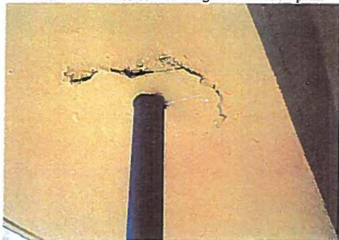
3. Plaster cracks
