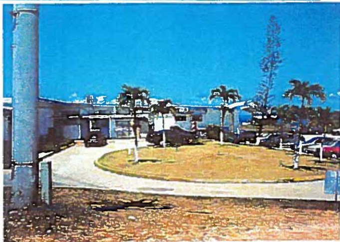
2. Side view of entrance
