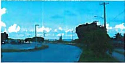
Overhead utility lines disrupt the ocean view.
