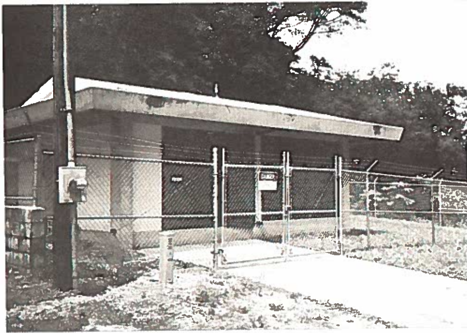
FIGURE 4-23 MALOJLOJ BOOSTER PUMP STATION
