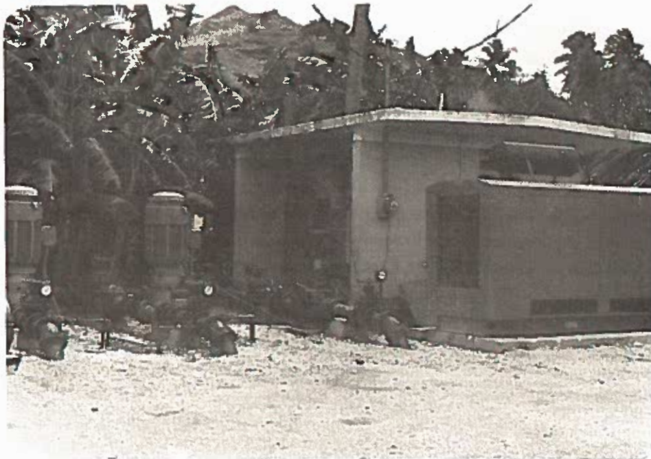
FIGURE 4-24 FIGUA BOOSTER PUMP STATION
