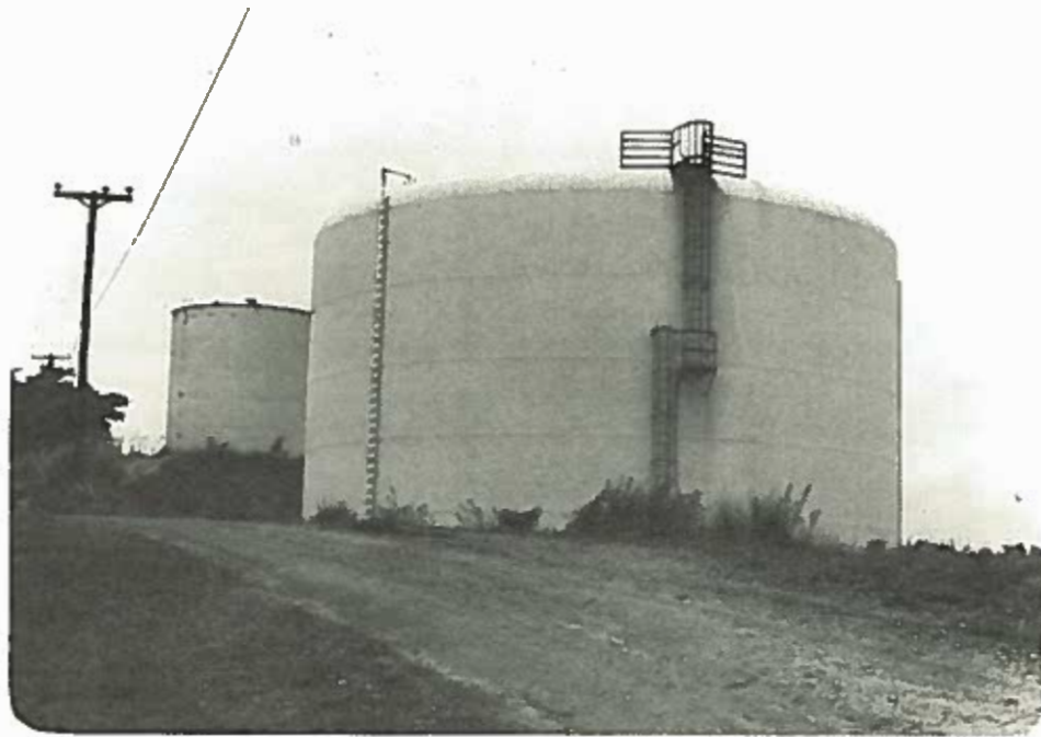
FIGURE 4-22 WINDWARD HILLS RESERVOIR
