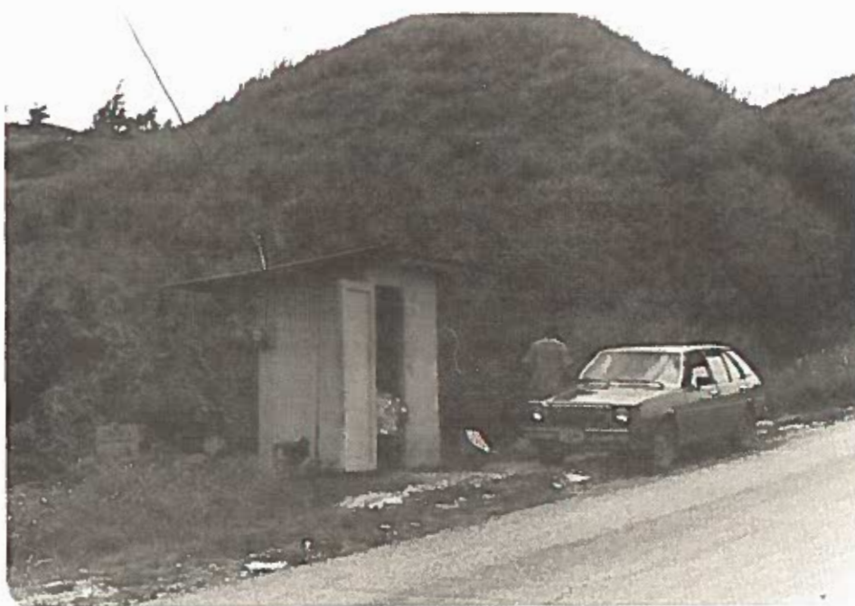
FIGURE 4-25 UMATAC BOOSTER PUMP STATION
