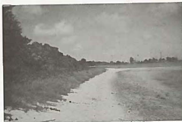
Typical View, Reach I
