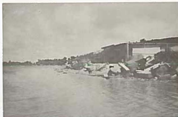
Typical View, Reach S
