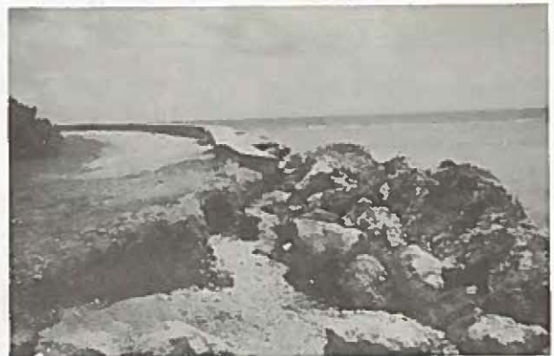
Severe Erosion, Reach L
