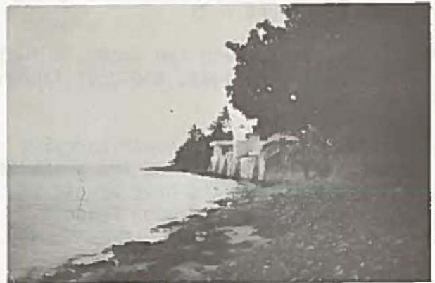
Seawall, Reach A
