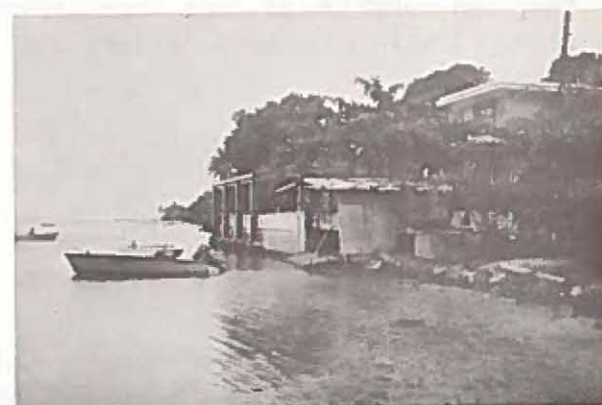
Rubble Seawall, Reach F
