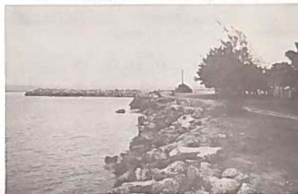
Revetment, Reach N
