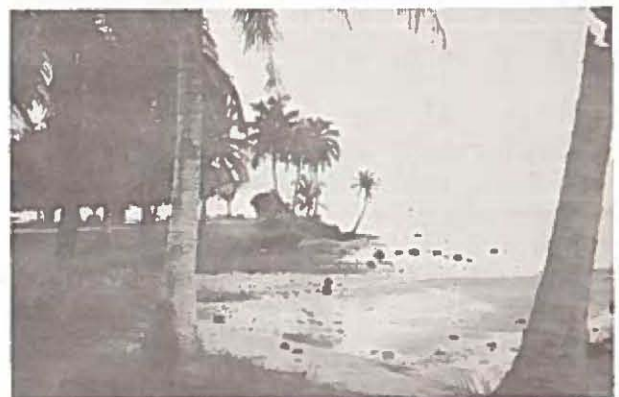
Erosion, North Side of Nimitz Beach Park
