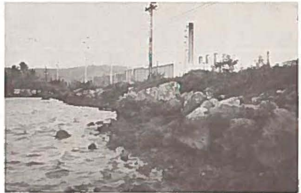
Revetment, Reach I
