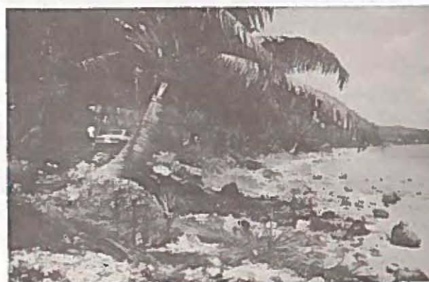
Minor Erosion, Trinchera Beach
