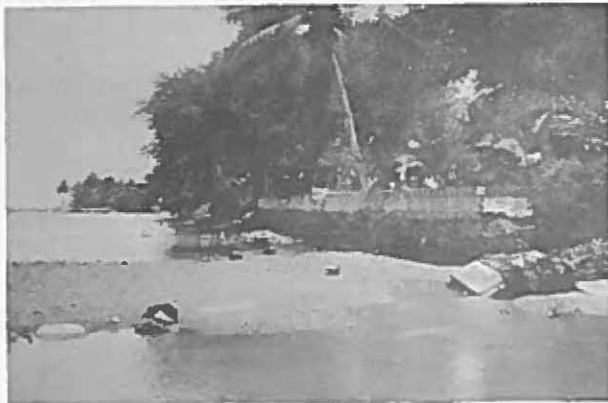
Grouted Seawall, Reach F
