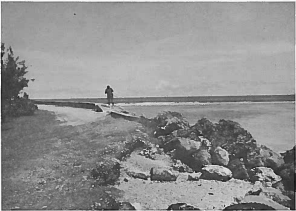
Photograph #1 East park shoreline near Station 3+00 looking north.
