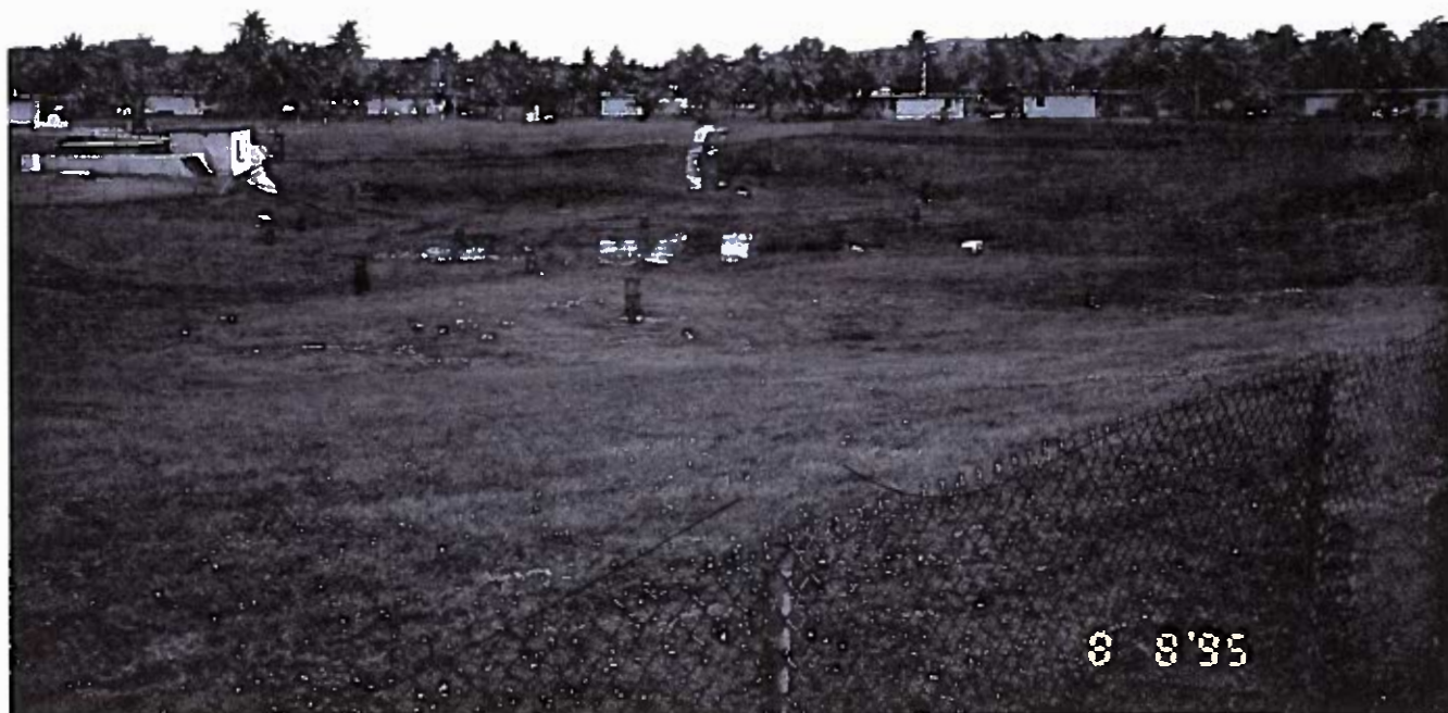
A2. Storm water drainage wells in housing area.
