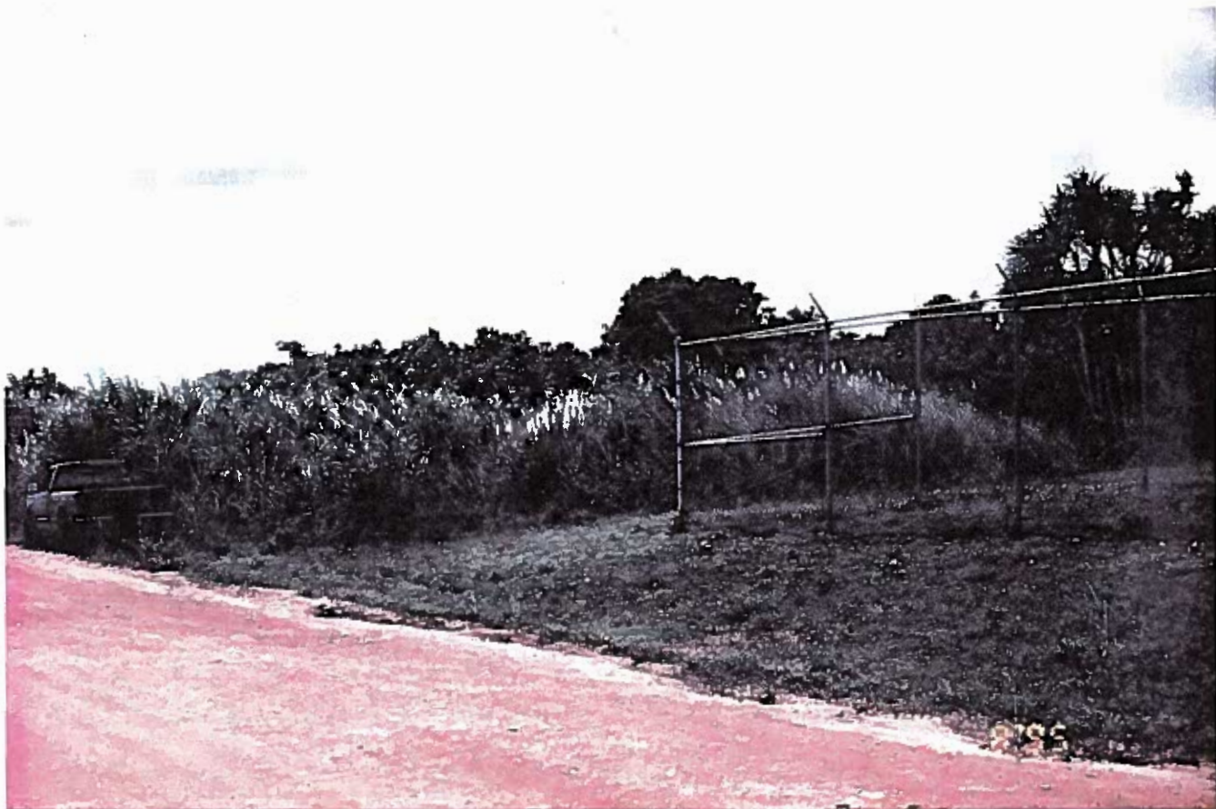
A1. S.W. corner of Landfill Cap, water diversion, with wildcane grass in background.
