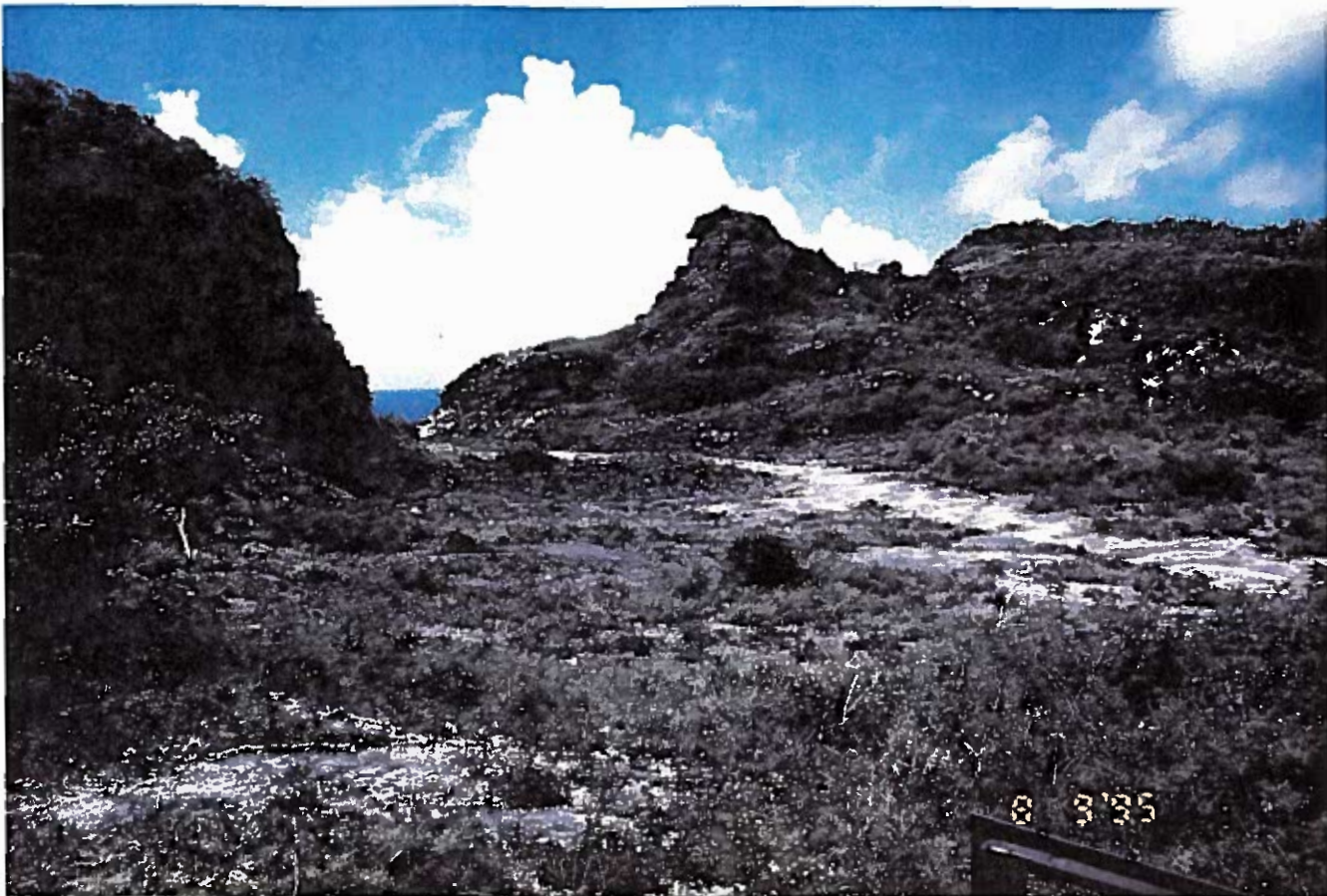
A3. Well drained Borrow Pit at Munitions Maintenance Area.
