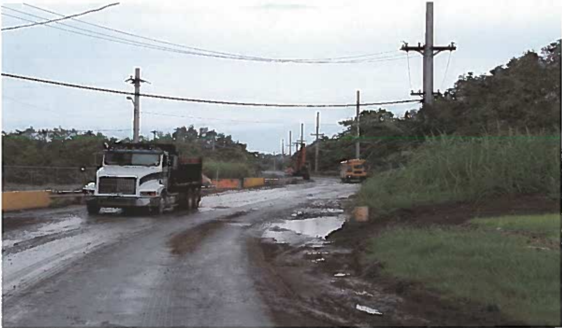
Merizo Road across from the Barcinas Compound experienced heavy flooding from low lying road.
