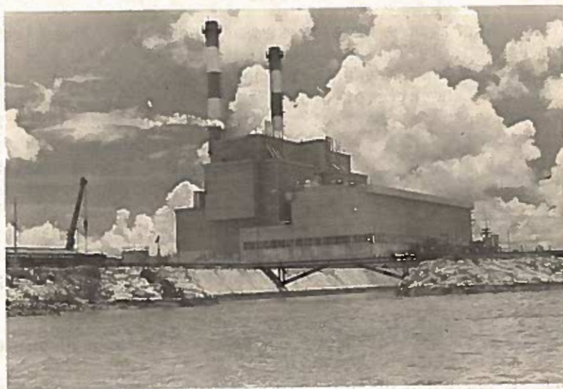
Figure 3. Cabras Power Plant with its outfall channel in foreground.
