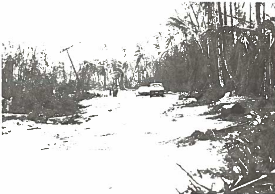
Destruction of Roads in Low-Lying Areas
