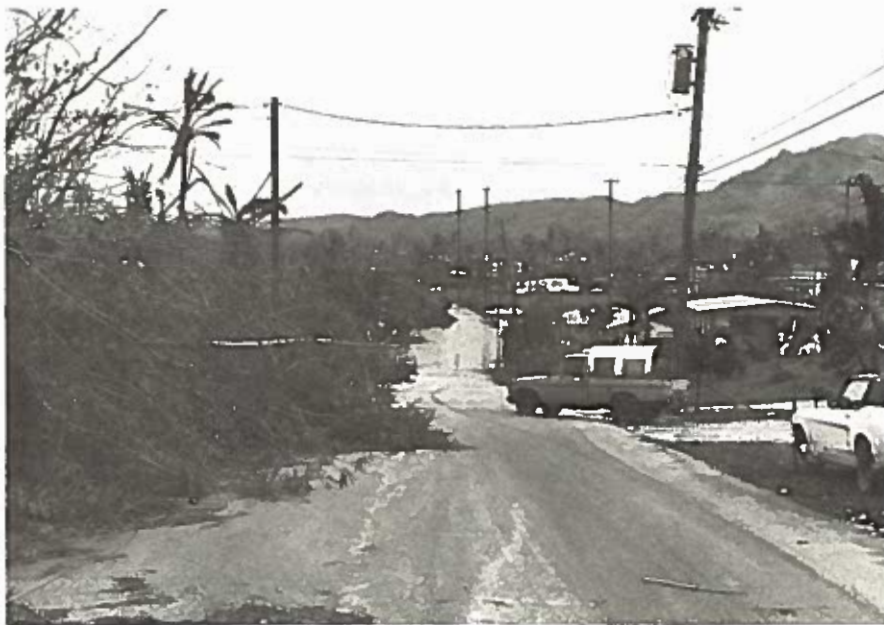
Flooding of Public Roads
