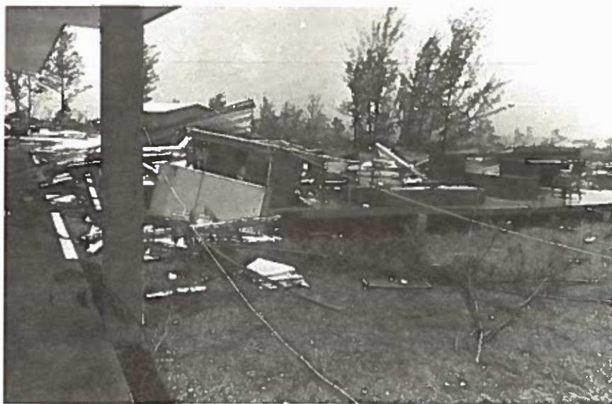
Destruction of Classrooms, Torres Elementary
