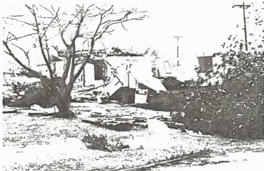
Residential Damage, Dededo
