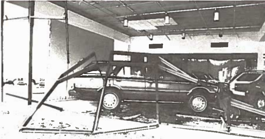
Commercial Damage, Tamuning
