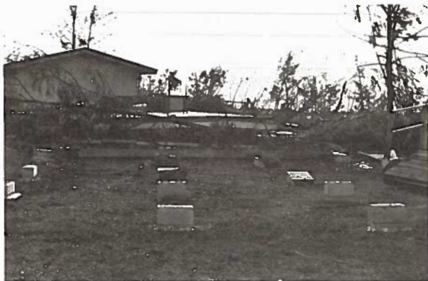
Destruction of Classrooms, Truman Elementary
