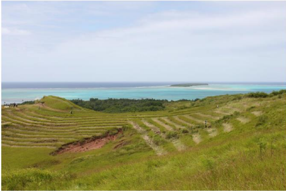
Site preparations in a High Priority Area.
