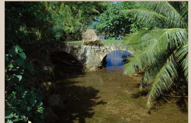
Taleyfac Spanish Bridge
