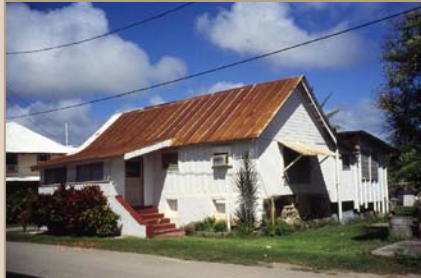
Mariano Leon Guerrero House before restoration
