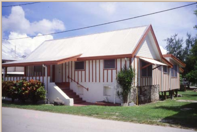
Mariano Leon Guerrero House after restoration
