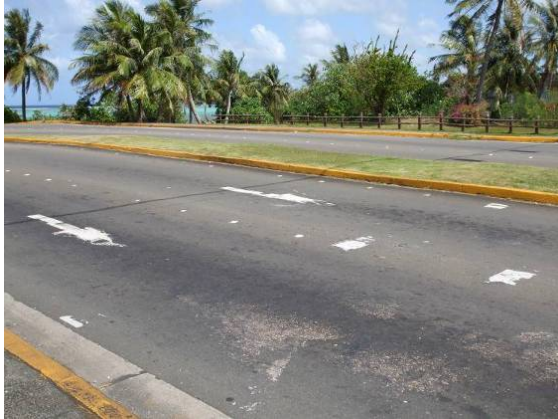
Figure 3-12: Sample Deteriorated Pavement Conditions
