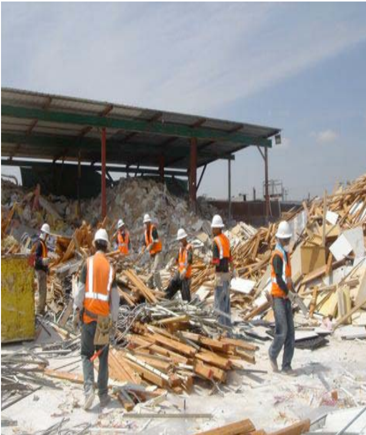
South Gate, CA C&D Facility (Interior Removal Specialists)
