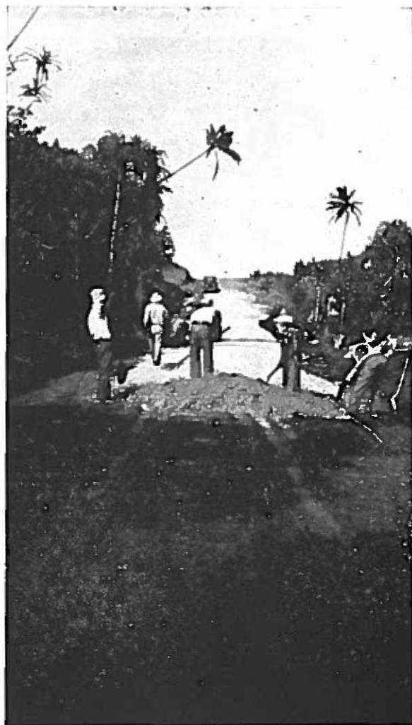
Spreading Cascajo—Fena Road
