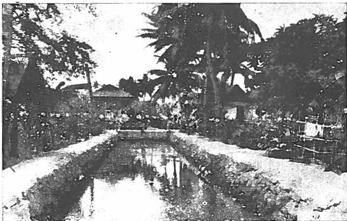
Santa Cruz Bridge west end of Agana River 1940
