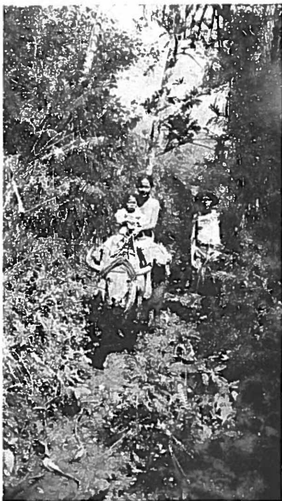
Fena Trail before Road was constructed
