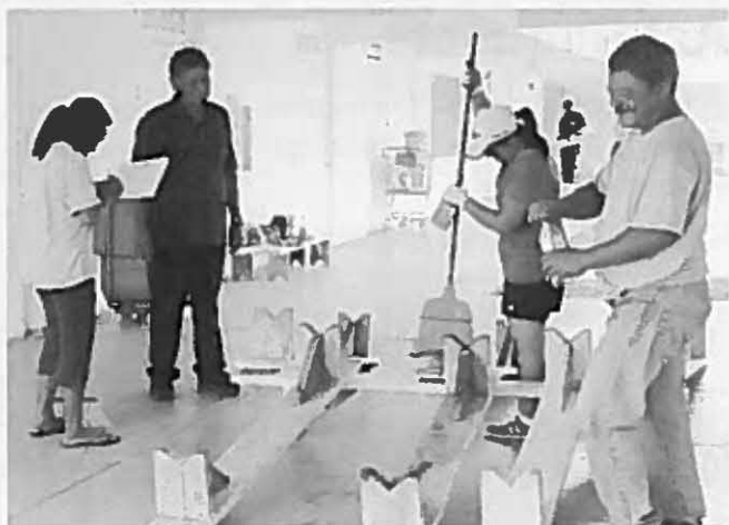
Preparing for school: Guam EPA helped B.P. Carbullido Elementary School get ready for the 2012-2013 school year. Guam EPA staff pitched in to waterblast, paint (above), fixing drainage issues and other work around the campus.
