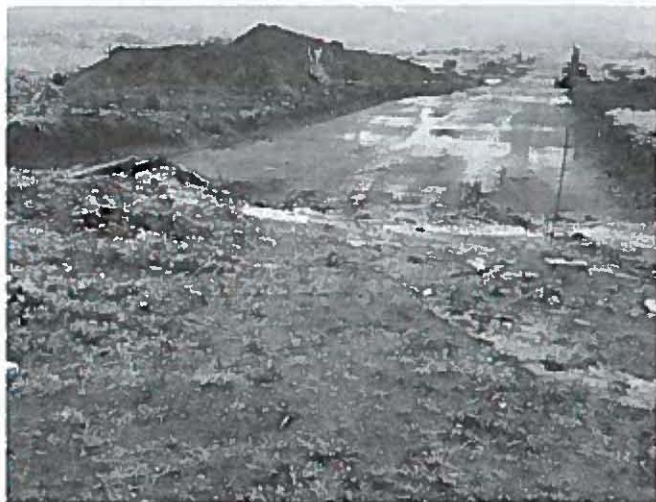
Clearing and Grading: The Water Pollution Control Program regulates different construction and clearing projects like the one below.
