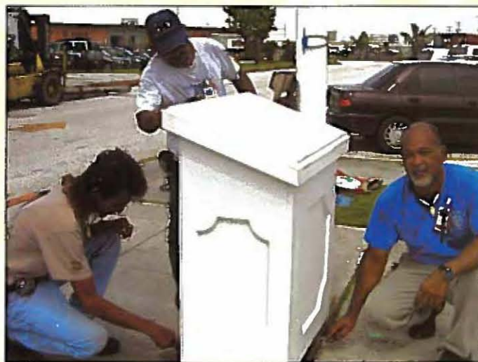
Employees from Facility Maintenance complete the memorial honoring Jose D. Leon Guerrero.
