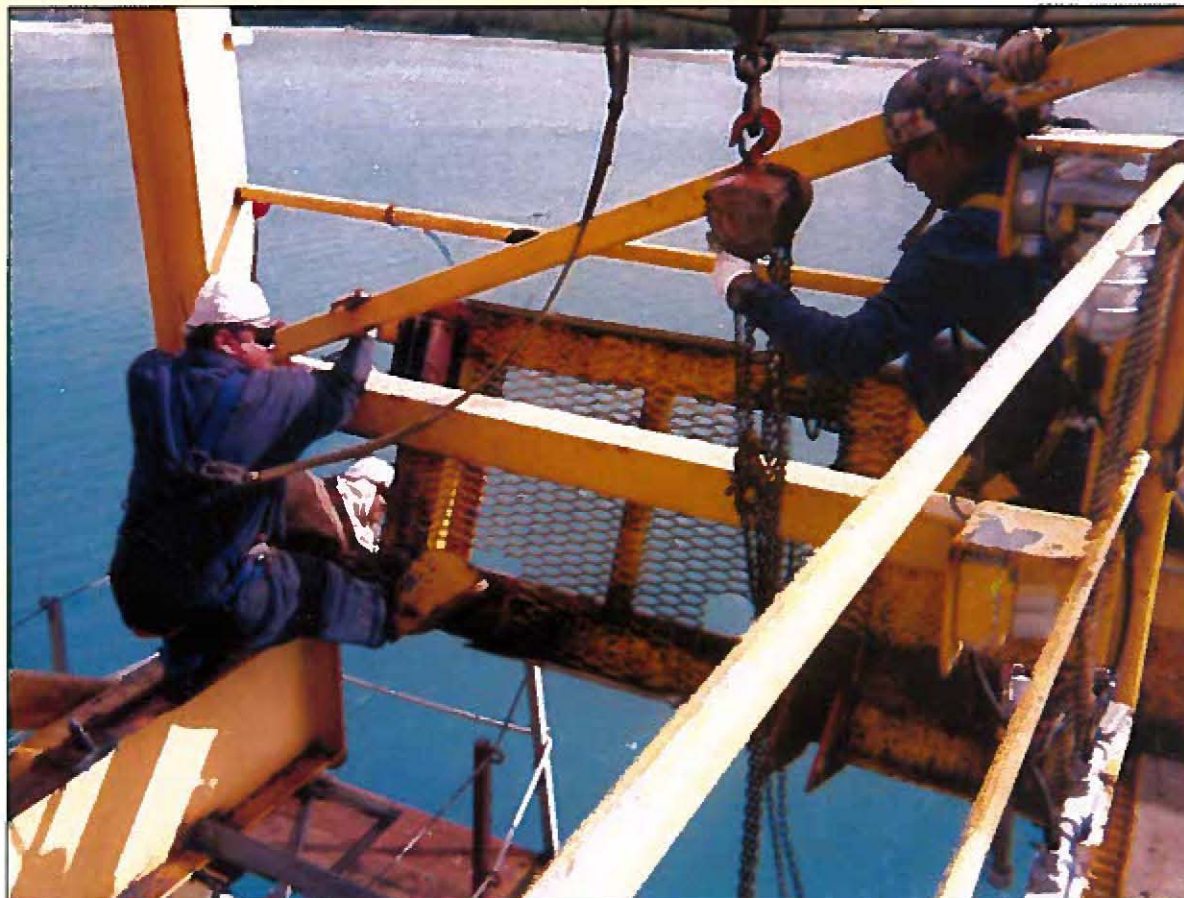
Welders performing routine maintenance on gantry crane.
