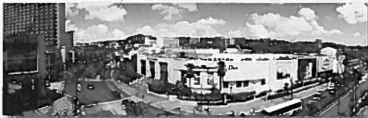
San Vitores Road Flooding Mitigation
