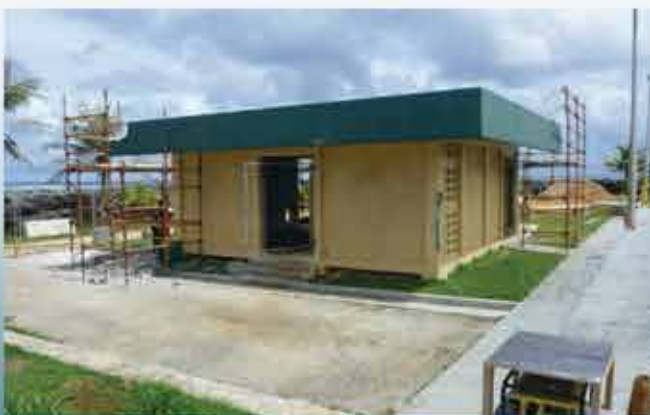
Hagåtña WWTP – Abandoned effluent pump room is converted into a chemical mixing and storage facility.
