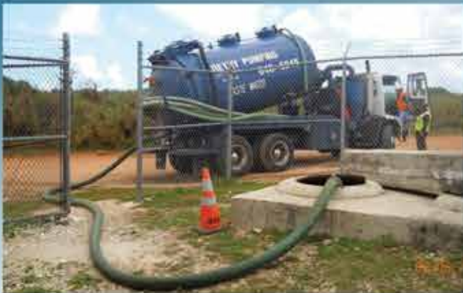
Northern WWTP Septage Receiving Station – Pre-construction dumping into a manhole ahead of the plant.
