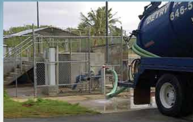
Post-construction disposal into a controlled facility that screens and equalizes Septage flow into the plant.
