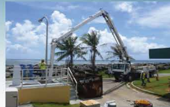
Hagåtña WWTP – Permanent closure of old outfall
