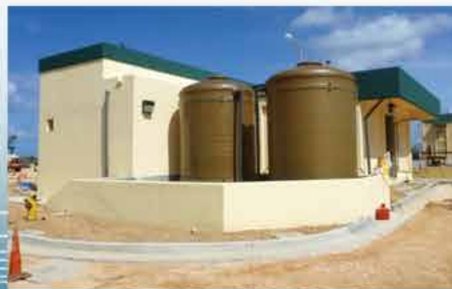
Hagåtña WWTP – Abandoned effluent pump room is converted into a chemical mixing and storage facility.
