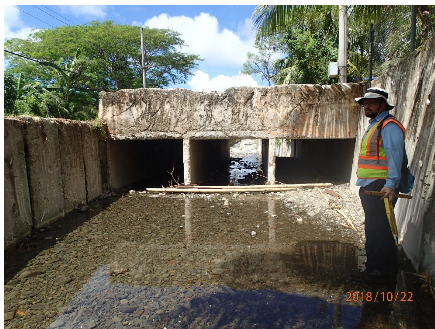
Photo 5-1: Bridge over Nelansa (Manell) River at XS 415
