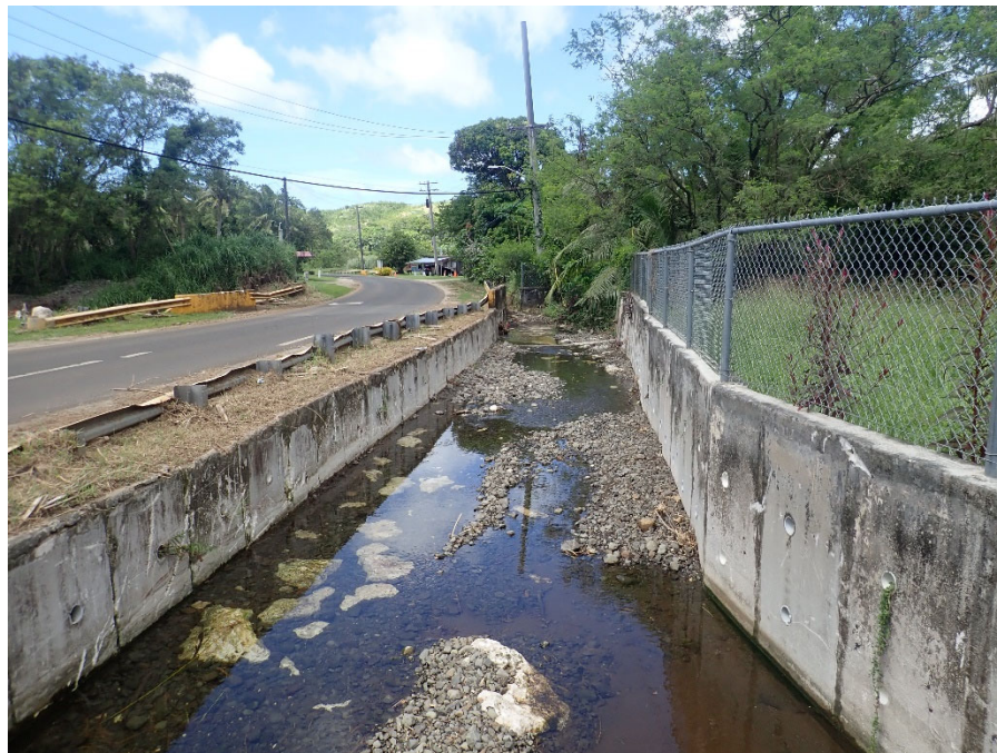
Photo 4-4: Tributary River, Concrete Ditch along Route 4
