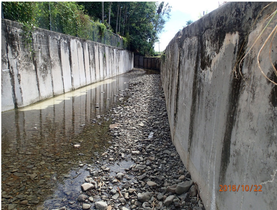
Photo 4-2: Nelansa (Manell) River, Concrete Channel Reach along Route 4
