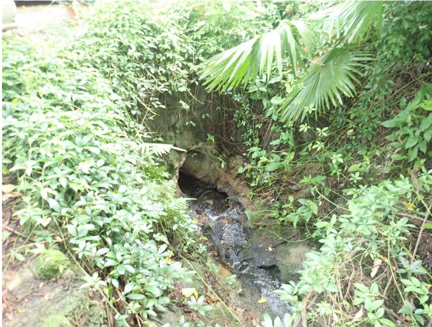
Photo 6-1: Road Culvert, October 2018
