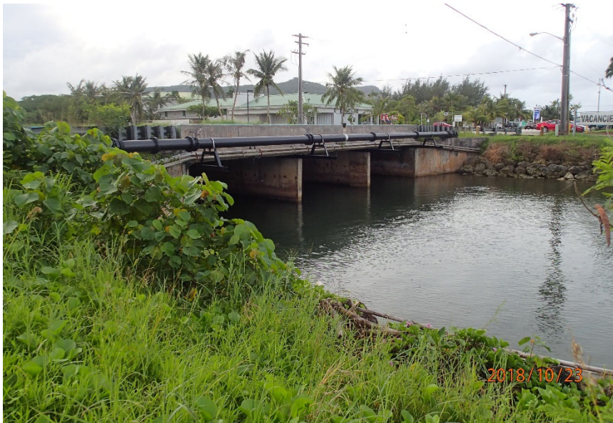
Photo 5-1: Looking upstream at the Highway 2 Bridge over Namu River at XS 120
