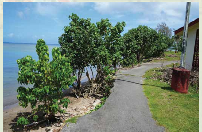
North facing view of the sidewalk and beach erosion at Nimitz Beach Park: facilities. (Photo by: Guam Coastal Management Program)
