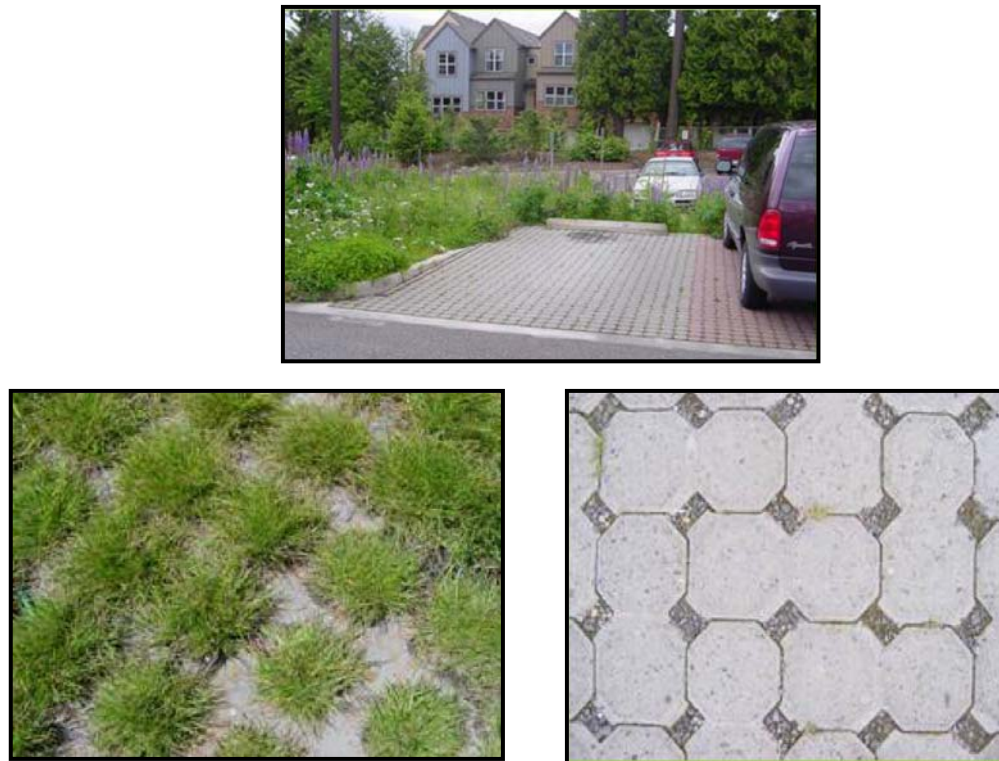
Figure 3.4 Examples of Permeable Pavers
