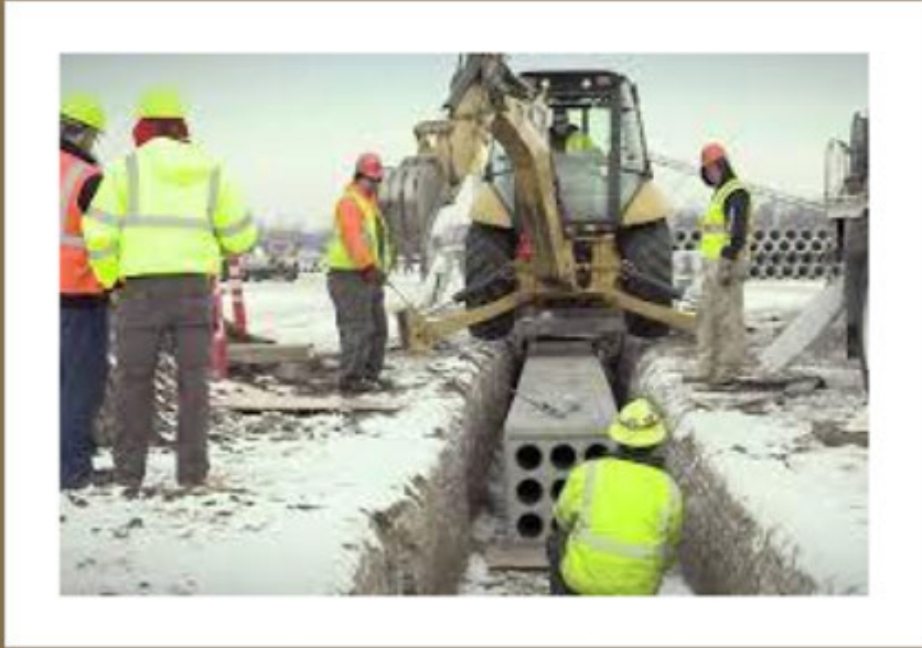
Marine Raceway Installation
