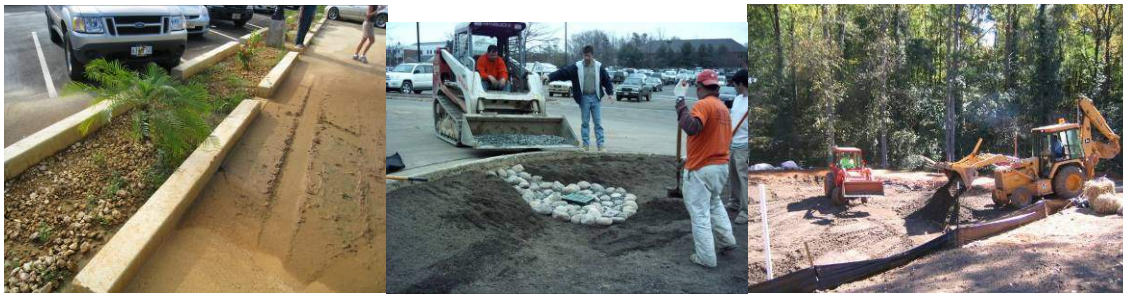
Figure S2.7. Construction sediment can easily damage bioretention filter bed (left). Block inlets during construction (middle) and/or install temporary silt fence around perimeter of bioretention during construction (right).
